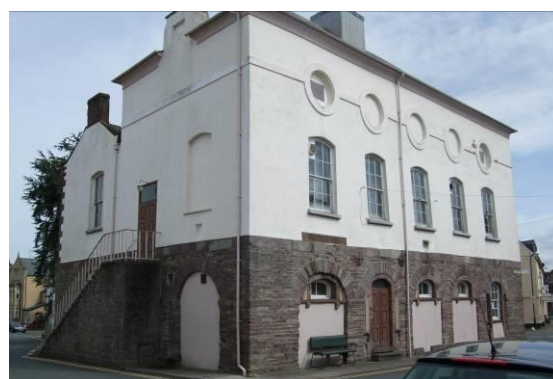
Fig.132 The Town Hall, south and west elevations. The ground floor arcading was infilled in the later 19 th century.
