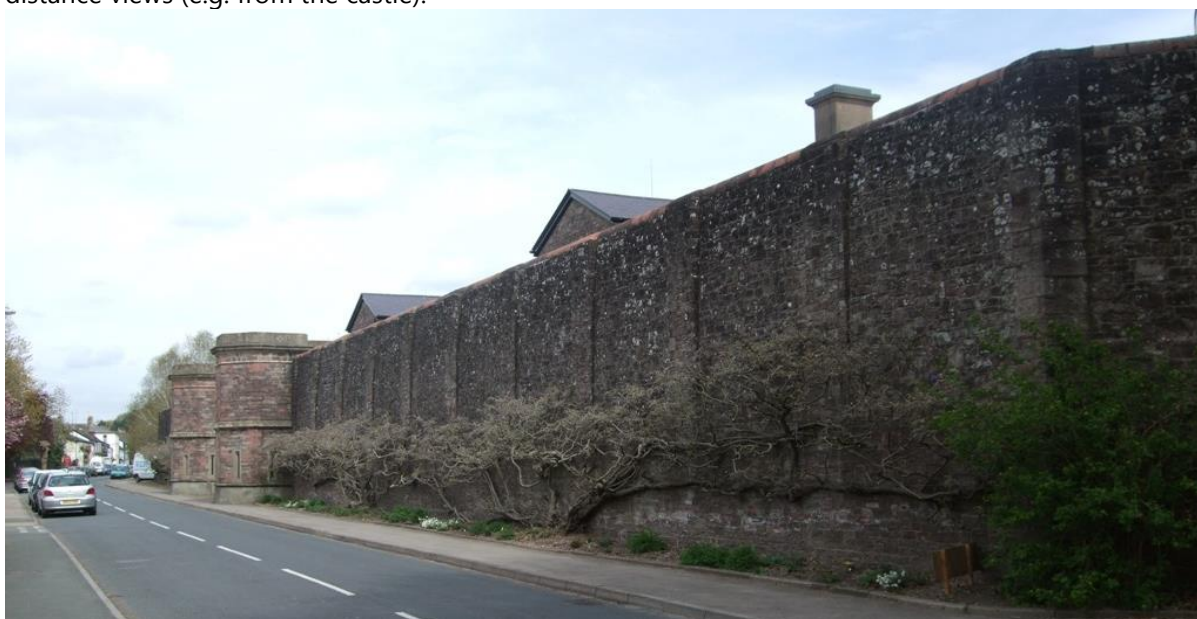
Fig.78 The scale and extent of the walls to the gaol fronting Maryport Street dominate the townscape to this part of the conservation area
