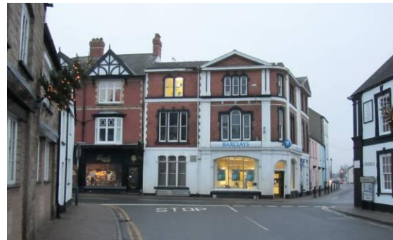
Fig.137 Barclays Bank, from Porthycarne Street
