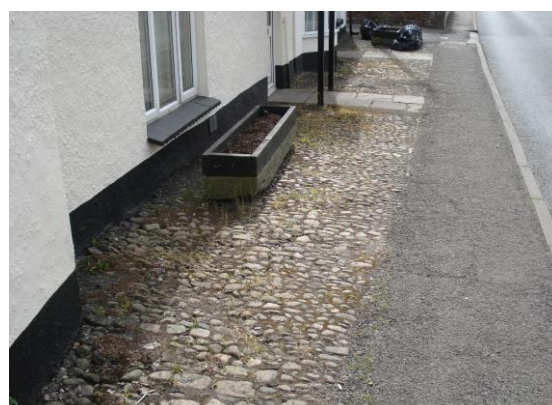
Fig.39 The historic use of cobbles for pavement finishes is an increasingly rare survival and significantly adds to the quality of the public realm within the conservation area
