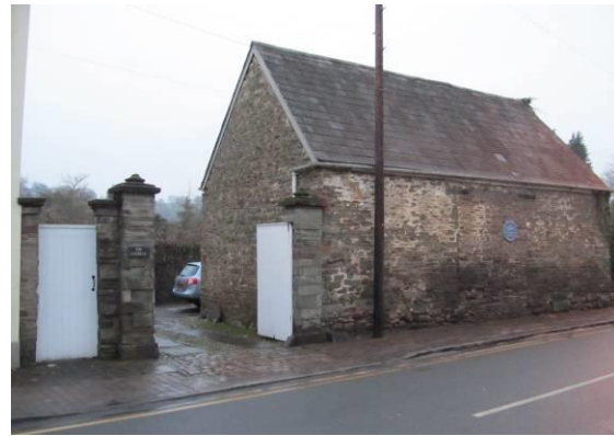
Fig.107 Former Barn in Porthycarne Street
