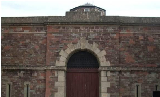
Fig.158 Squared stone to Usk Gaol
