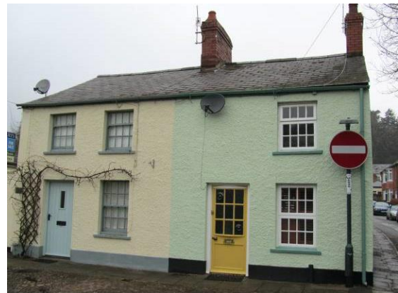
Fig.121 Cottages at the corner of Four Ash Street and Castle Street.
