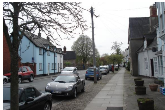
Fig.72 A bolder use of colour is seen to this part of the conservation area –particularly Maryport Street
