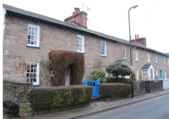
Fig.116 Fine late 18 th century terraced cottages, Baron Street.
