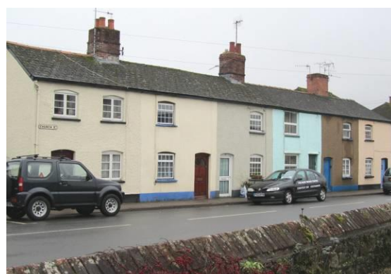
Fig.114 Early 19 th century range of cottages, Church Street.
