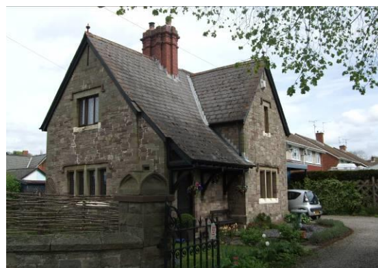
Fig.143 Priory Lodge, Maryport Street
