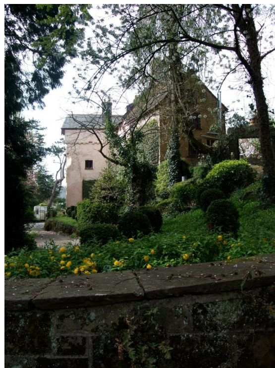
Fig.60 The Gatehouse and Castle House to the south-east of the remains of the Inner Ward, Usk Castle. The house is clearly seen from the public footpath through dense vegetation due partially to its scale and partially to its use of coloured limewash
