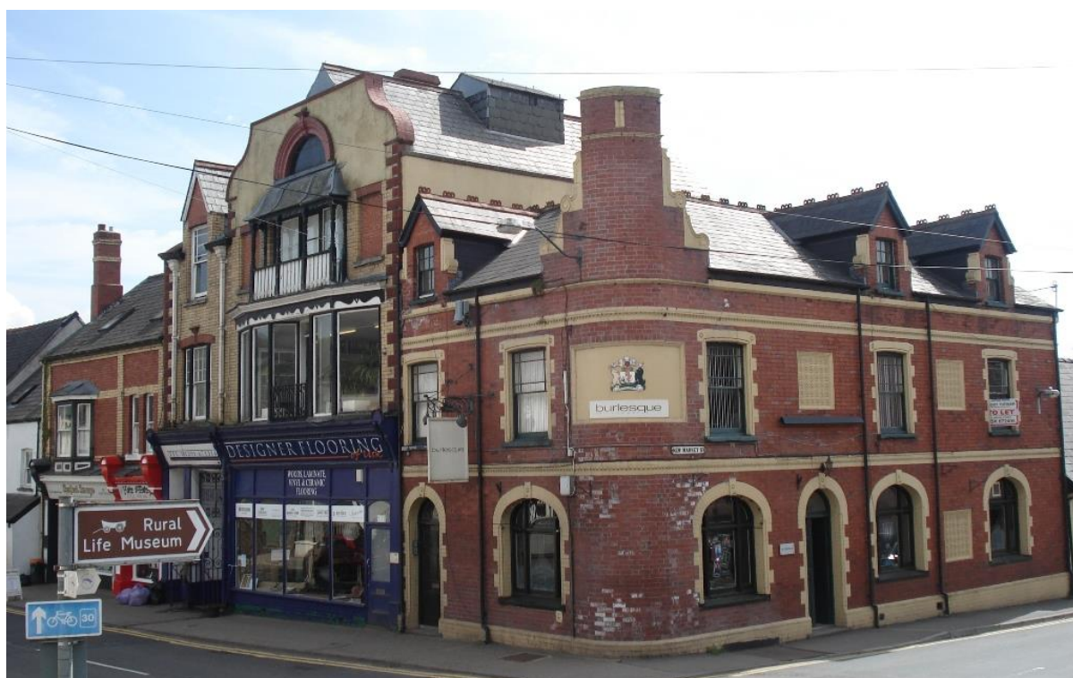
Fig.20 The distinctive use of red and buff brickwork on prominent buildings in the street scene – pictured No.69 Bridge Street
