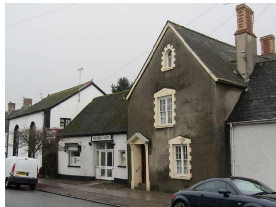
Fig.110 The Old Smithy (centre), Maryport Street
