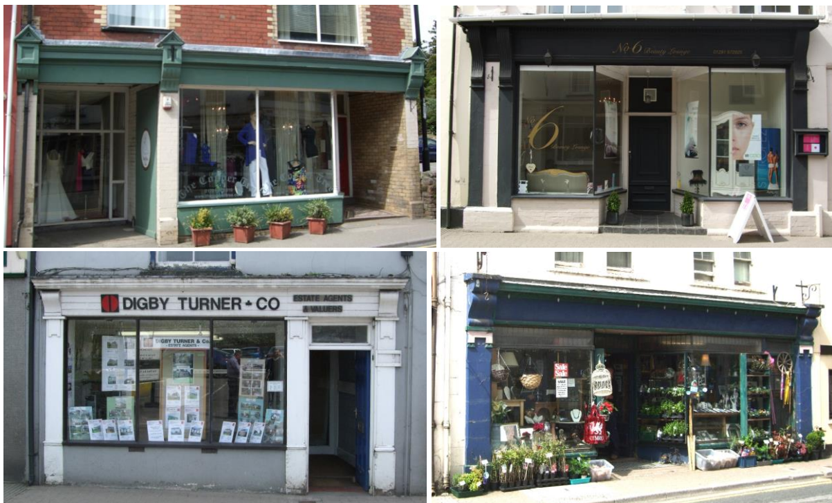
Fig.24 A sample of traditional shopfronts in Bridge Street.
