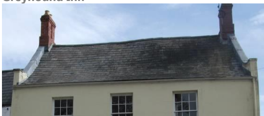
Fig.162 Natural slate is still seen to traditional buildings, often behind parapets
