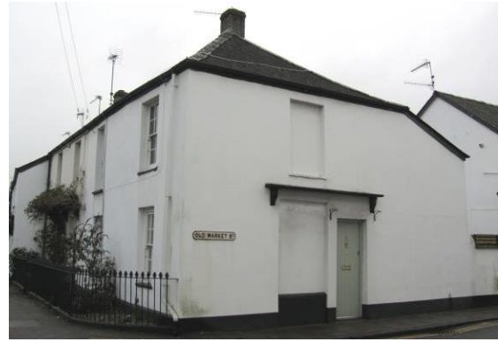
Fig.119 Corner building Old Market Street and Maryport Street.
