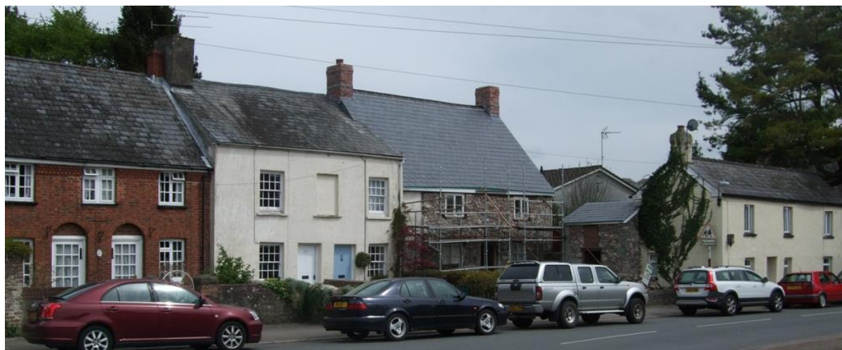
Fig.67 An attractive group of vernacular cottages to Four Ash Street
