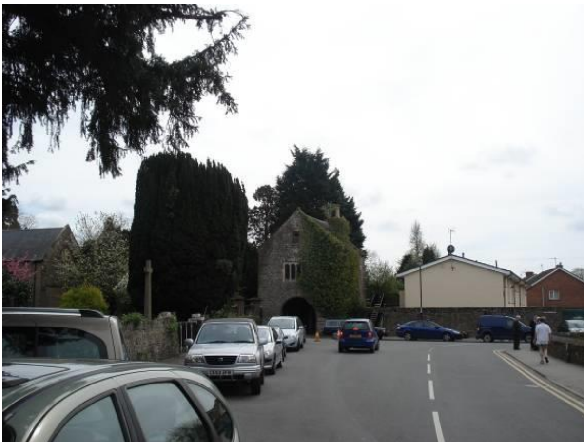
Fig.70 The space forming the junction of Church Street and Priory Street is well-defined by the Priory Gatehouse and the Churchyard wall
