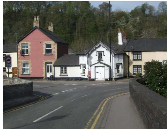
Fig.84 The view west across the bridge from the town is closed by the wide canted bay and gable of the former turnpike toll house, Woodside
