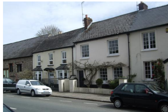
Fig.35 Roofs are generally natural slate with a number of attractive groups of uninterrupted roof slopes such as these houses to the east side of New Market Street
