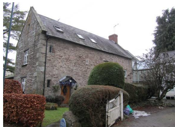
Fig.96 The former Guest House for the Priory
