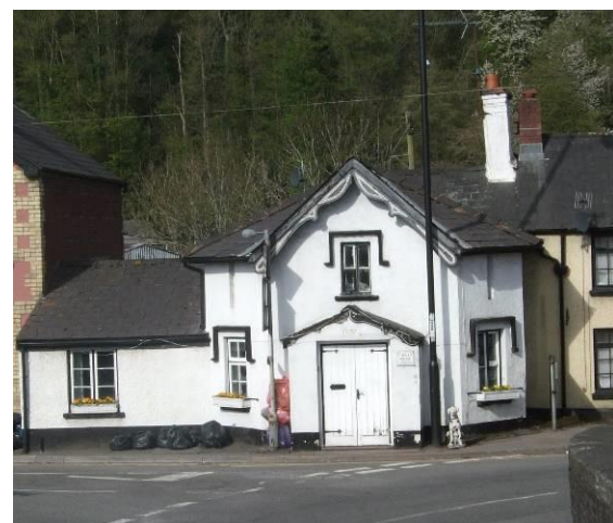
Fig.140 The Old Toll House on the west side of the Bridge.
