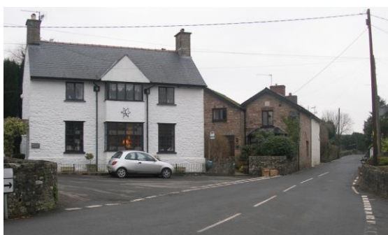
Fig.54 Newton Lodge: another Vernacular Revival house c1907, whose simple symmetrical design effectively terminates views in the village centre
