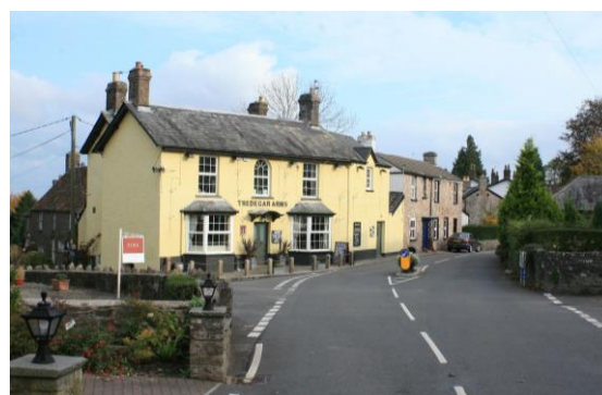
Fig.12 Tredegar Arms: positioned on a key corner site in the centre of the village
