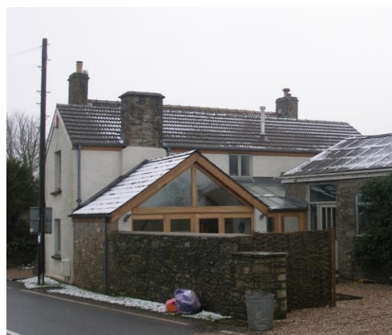
Fig.57 A contemporary and sensitively designed rear extension to a cottage near the playing fields – its appropriately subservient form enhances the original building
