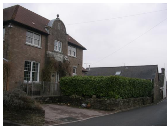
Fig.55 The former Police house of 1911: its semi-circular gable, paired sash windows and buttresses flanking the entrance distinguish this simple building
