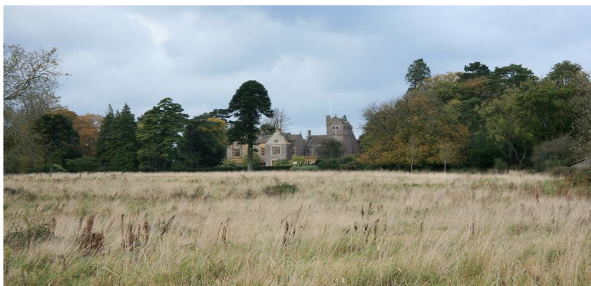
Fig.39 Shirenewton Hall seen across the rough pastureland to the south-west
