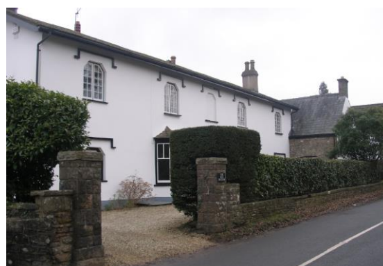
Fig.49 The Old Rectory: an elegant five bay late Regency house with interesting canted window heads. A remodelling (conversion from three estate workers dwelling according to the list description)
