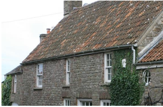
Fig.17 Attractive combination of coursed rubble stone and clay pantiles to the Old Meeting House
