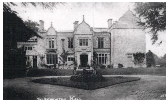
Fig.6 Shirenewton Hall c.1907
