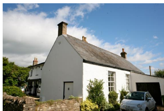
Fig.62 Natural slate roof to the Old Rectory
