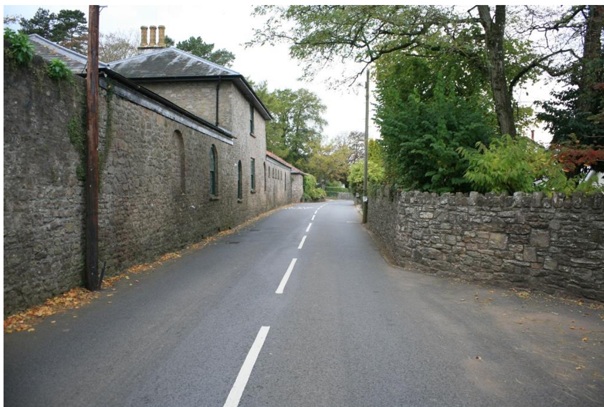
Fig.21 High stone walls and integrated outbuildings strongly define the boundary to the grounds of Shirenewton Hall
