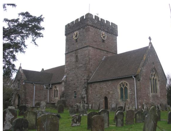
Fig.47 St Thomas à Becket church: its solid battlemented medieval tower contrasts with the largely restored Victorian chancel and nave
