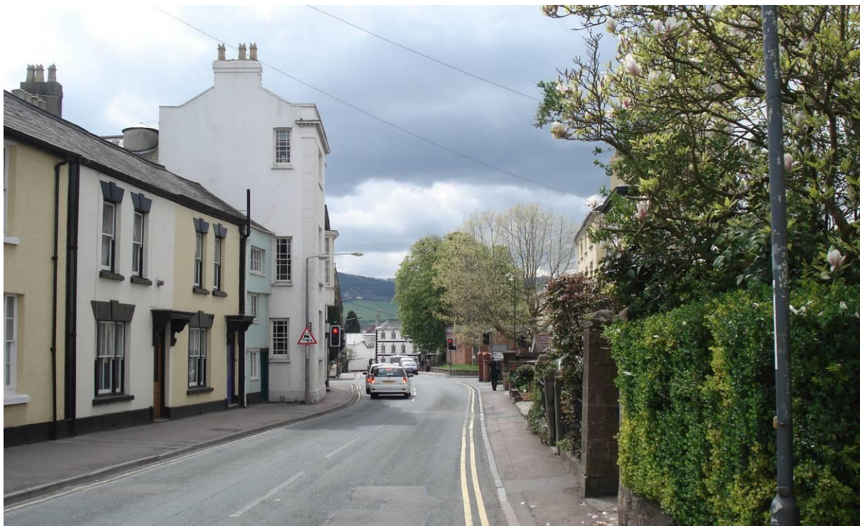
Fig.93 View looking south along North Parade into Monk Street, note the green backdrop to Whitecross House seen in the distance closing the vista along Monk Street
