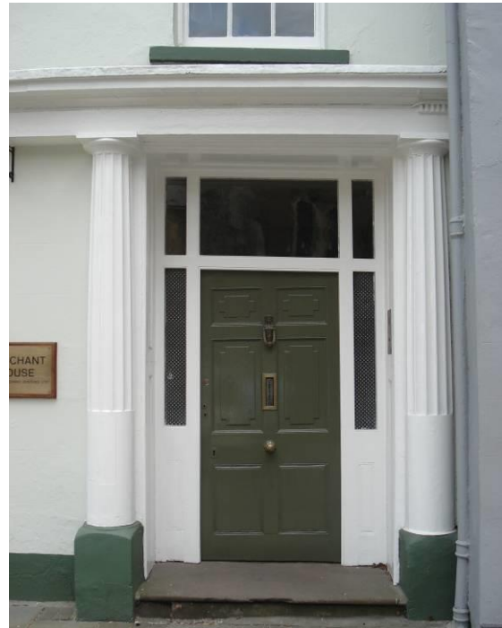
Fig.42 One example of the many grand doorcases found in the character area
