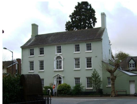
Fig.81 Overmonnow House opposite the church, one of several large townhouses which dominate the street scene with their scale accentuated by the symmetry of the built form and the emphasis of the upper storeys, in this case with the use of a central arched window with moulded architrave
