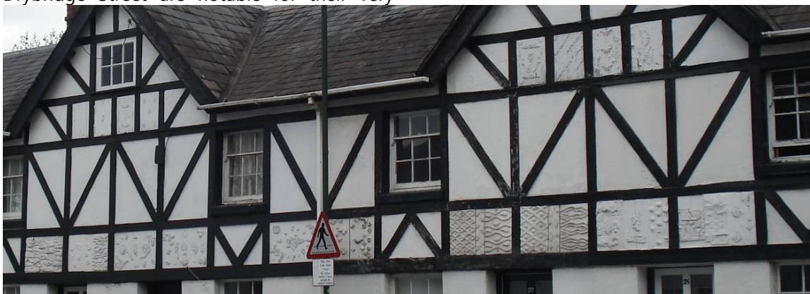
Fig.92 Drybridge Street houses displaying an unusual decorative motif created with wallpaper manufacturer's blocks
