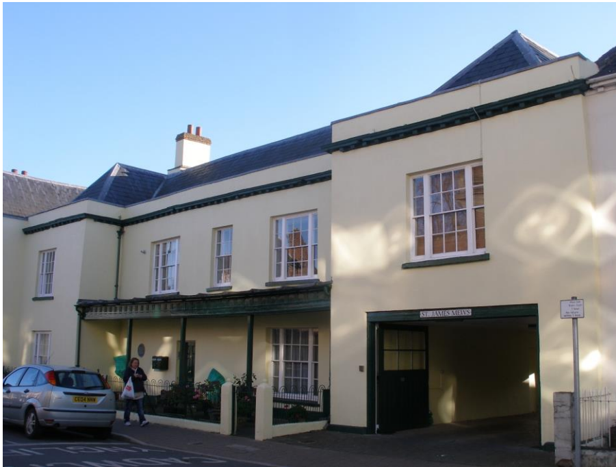
Fig.114 Nos 1 & 2 Whitecross St. 16 th century origins although refronted and reroofed in the 18 th and 19 th centuries.
