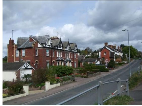
Fig.204 19 th century terrace on Hereford Road
