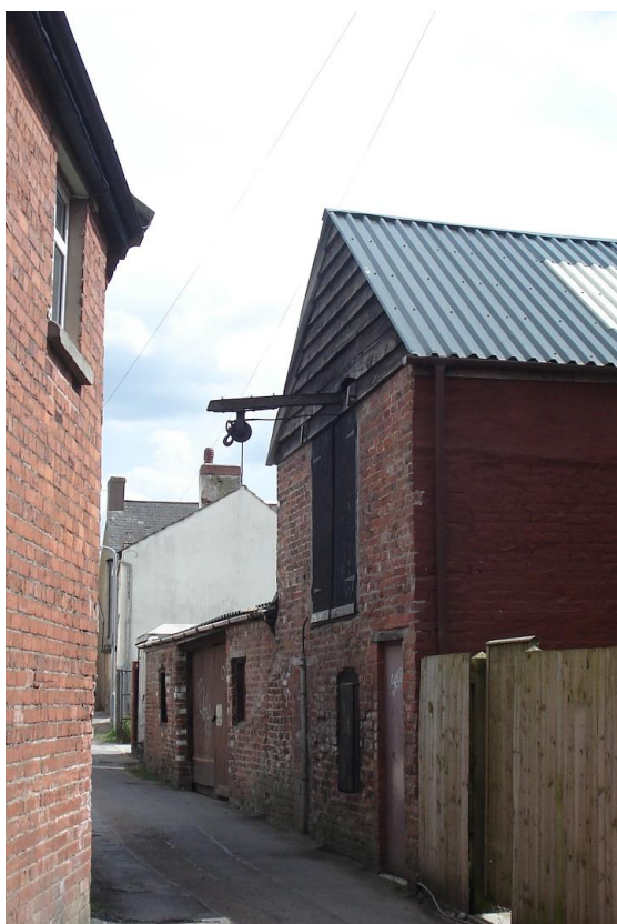
Fig.56 Small warehouse/store building – south side of Nailers Lane
