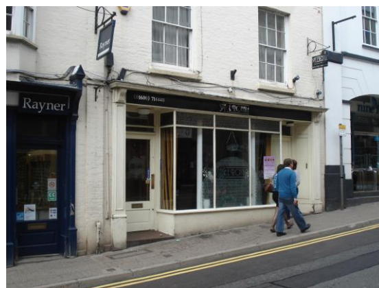
Fig.60 Shopfronts and signage to Monnow Street are generally of a good quality, using traditional materials. Hanging signs in particular are modest in scale and are not overbearing
