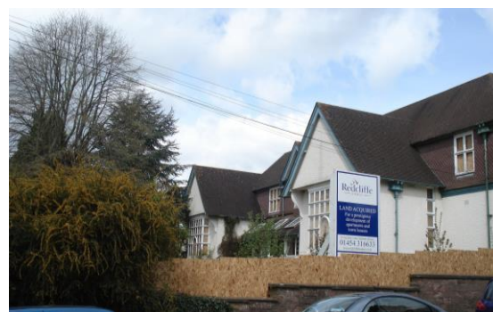
Fig.75 The former cottage hospital (presently vacant and in a poor condition – Oct 2010) is set into the hillside and has two prominent gables facing out to the town
