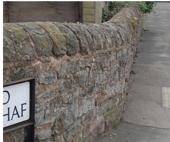
Fig.90 Boundary walls within the conservation area incorporate local stone with a distinctive half round capping
