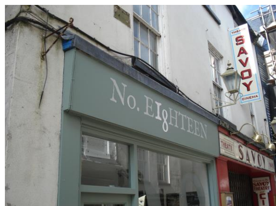
Fig.24 Simple, restrained and well-designed shopfront and fascia. The font and design of this signage is particularly successful
