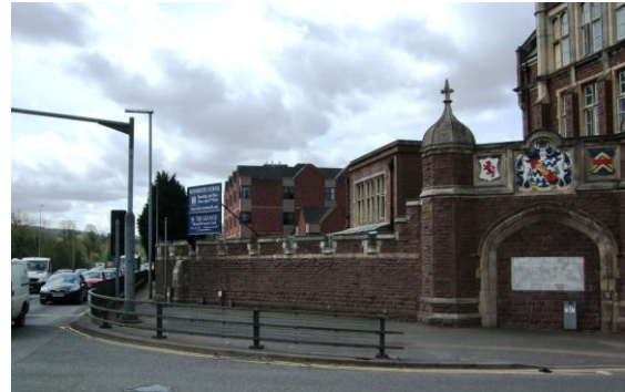
Fig.65 The stone boundary wall to the east side of the school site maintains the historic line of the extent of the schools grounds. A footpath to the river bank has been replaced by the A40 effectively forming a bypass for Monmouth
