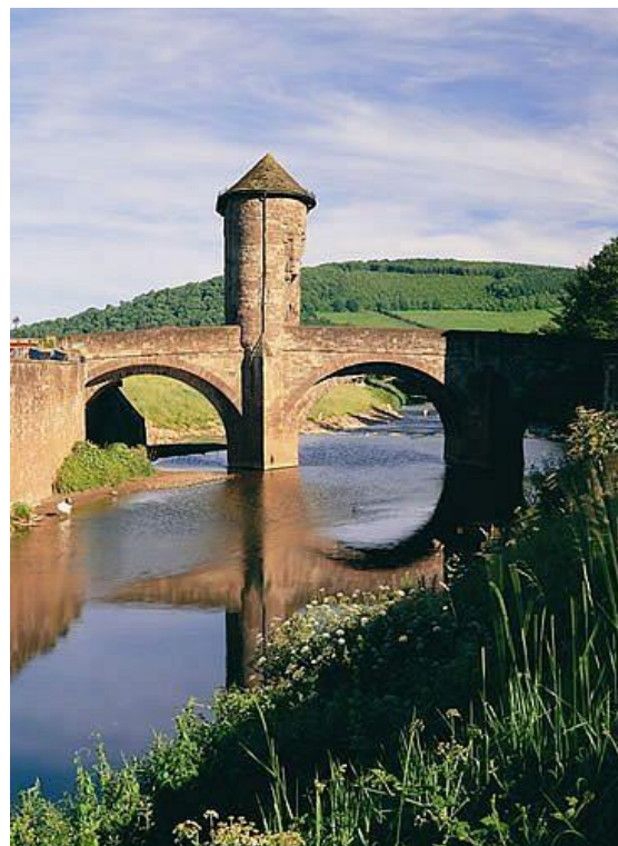
Fig.61 The gate house sitting astride the bridge – an important landmark to the southern end of Monnow Street
