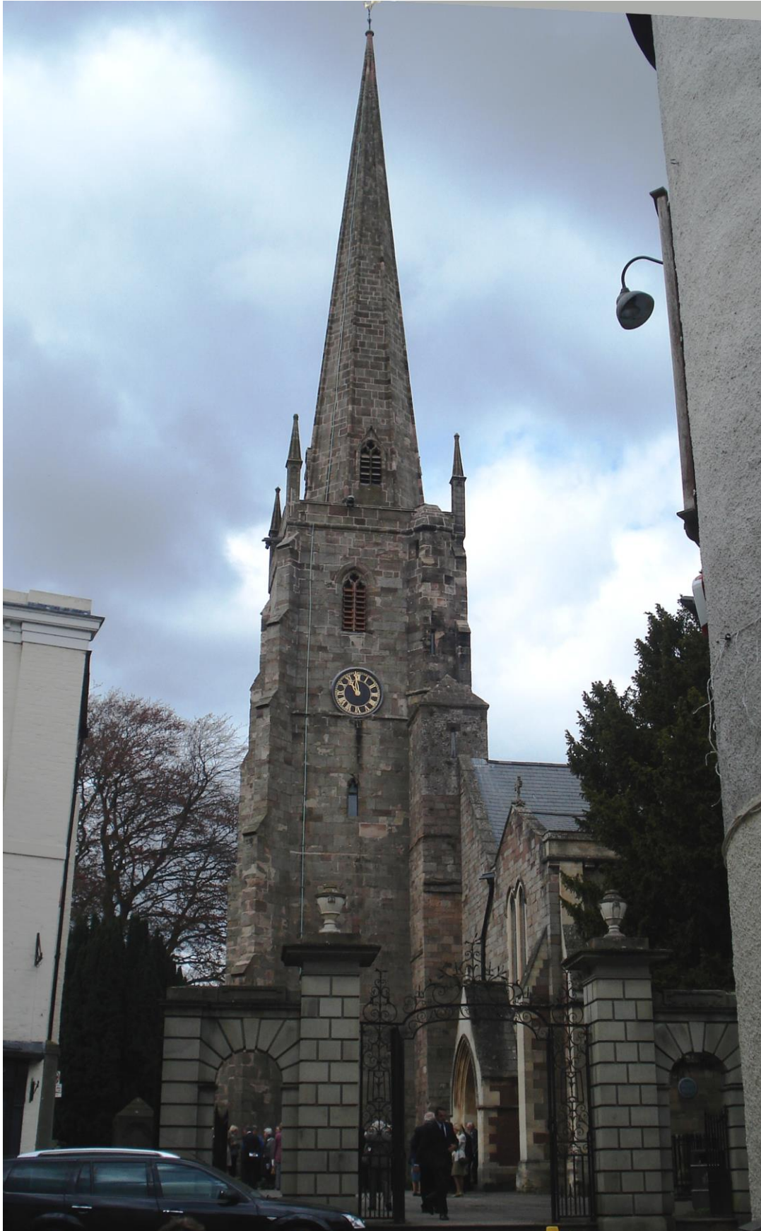
Fig.36 The gates, screen and gate piers to St Mary's church are an important local feature in the street scene
