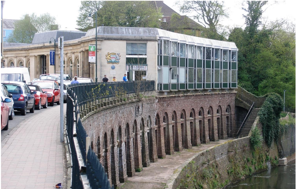
Fig.138 The massive retaining walls and arches housing the Shambles, with the former Market Hall at street level. The extent of the rebuild of the 1960s is evident from this view.
