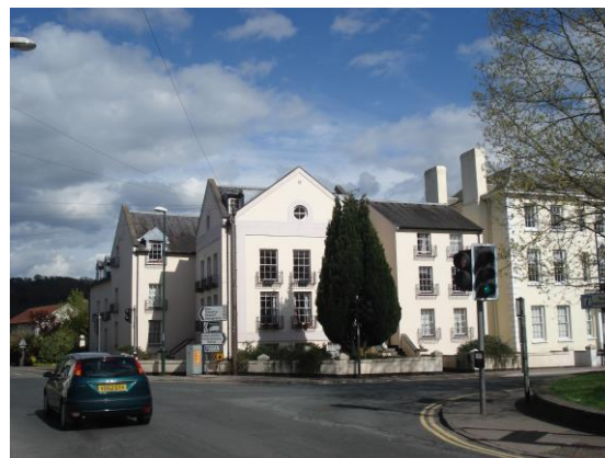
Fig.101 New buildings to the junction of Monk Street and Dixton Road maintain the important enclosure to this junction and building line to these major routes
