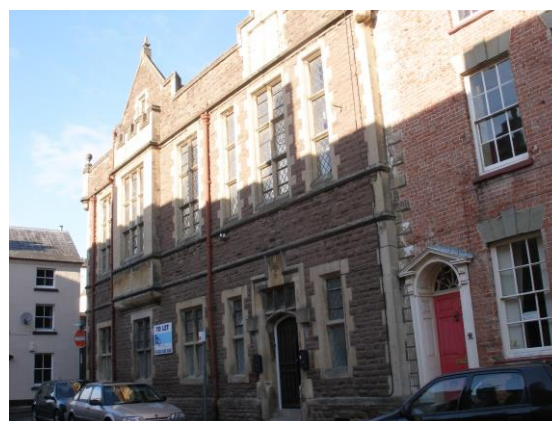
Fig.153 The Nelson Rooms, on the corner of Glendower Street and Agincourt Street continues the theme of institutional buildings designed in the Gothic Revival style and constructed in red sandstone with Bath stone dressings.
