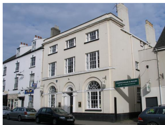
Fig.127 Chippenham House, Monnow Street, a late 18 th /early 19 th century house whose low pitched roof is typically hidden by a parapet.
