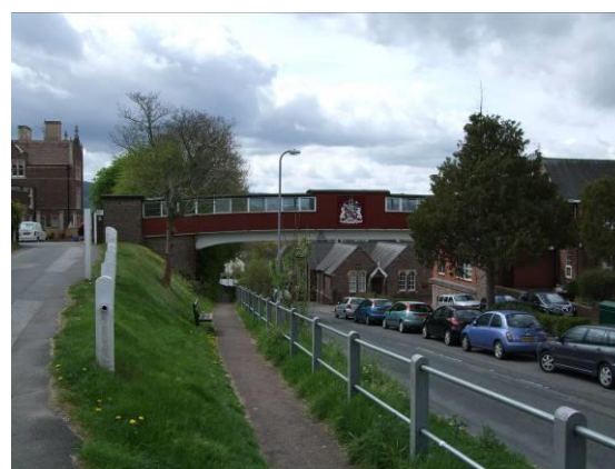
Fig.72 The pedestrian bridge linking school sites either side of the Hereford Road and acting as both local landmark and informal gateway to the town from the north
