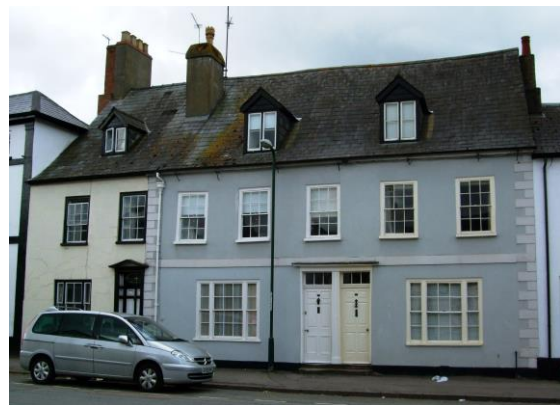
Fig.85 A subtle variation in the use of colour tone adds to the character of the streetscene and accentuates the architectural qualities of the buildings
