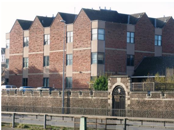
Fig.175 The Science Block of the Boys' School, of 1981, makes reference to the gables and red sandstone of the original buildings, whilst being a building of its time
