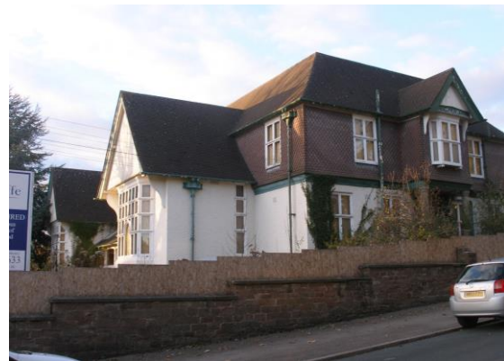
Fig.170 The extensive former cottage hospital building, set at right angles to Hereford Road, dated 1903. Its simplicity, massive mullioned and transomed bay windows and sweeping gables mark this as a relatively rare and high quality example of the Arts and Crafts style in central Monmouth'.
