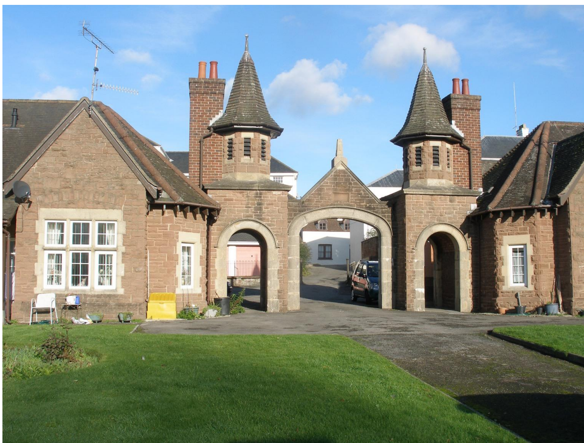
Fig.172 Henry Burton Court almshouse group, whilst built in 1928 has distinctively Victorian characteristics
