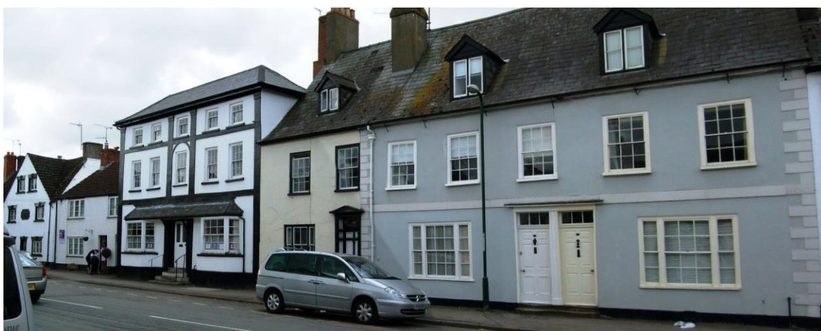
Fig.79 The townscape of Overmonnow is characterised by its diversity; varied roof forms, heights and use of materials. It is a townscape borne out of the adaptation and remodelling of buildings over time to produce a patina of age which is very difficult to reproduce
