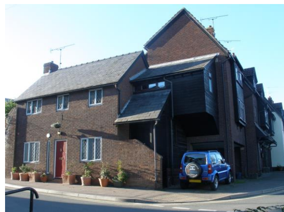
Fig.177 The Burgage, c1980s, an interesting handling of a tight corner site off Dixton Road, to create a higher density housing scheme
