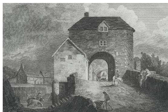
Fig.5 Monnow Bridge with its fortified gatehouse, J Varley, 1801
