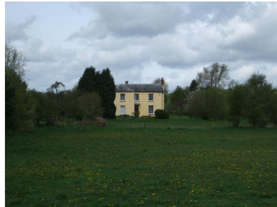
Fig.107 Vauxhall Farmhouse a prominent Grade II listed building clearly seen in extended views from the town and from across the floodplains.
