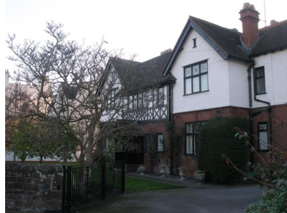
Fig.169 The Gables Hereford Road, one of a handful of spacious houses of the Domestic Revival dating from the turn of the 19 th /20 th centuries.
