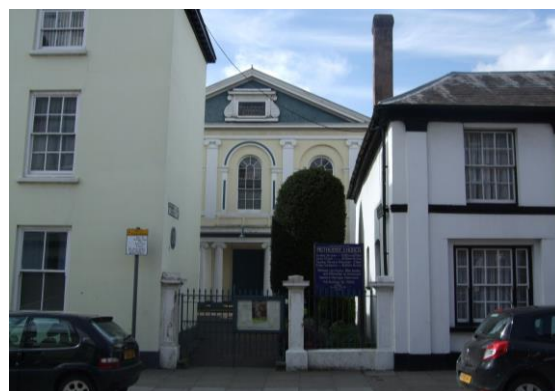
Fig.39 Monmouth Methodist church set back from the street line is dramatically accessed via a gap between houses which has been designed as a small forecourt which gives the well considered classically inspired façade some modest sense of a setting
