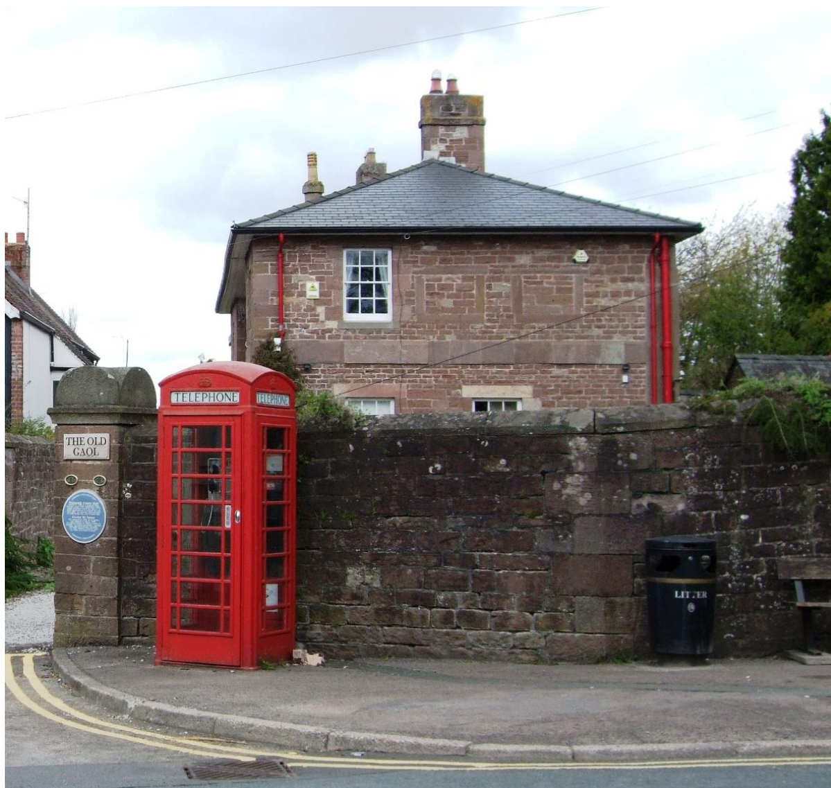
Fig.102 The gatehouse to the former County Gaol. The use of Old Red Sandstone blocks clearly defines the original window configuration on this building. The Gaol Gatehouse and its high stone wall form a good group
