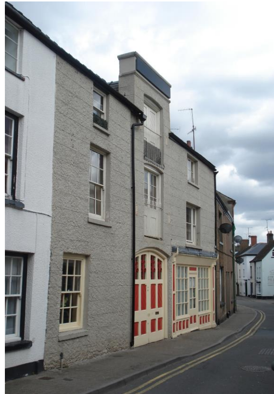
Fig.20 This building in St Mary's Street has had a variety of uses with the features such as the carriageway arch and shopfront adding to the special character of the street and breaking up the street scene
