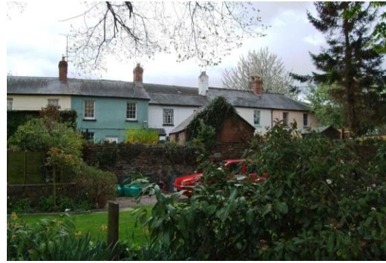
Fig.80 Drybridge Terrace – an attractive group of modest terraced houses set perpendicular to Drybridge Street and seen in the setting of their front gardens from Drybridge Terrace
