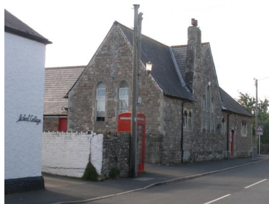
Fig.58 The 'Old School' on the main road is of a typical Victorian Gothic Revival design with steep pitched roofs, gables and ecclesiastical style details and windows
