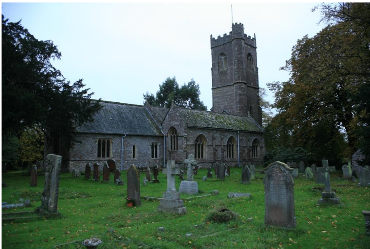
Fig.15 The church displays a harmonious palette of materials comprising limestone and sandstone with ashlar tower
