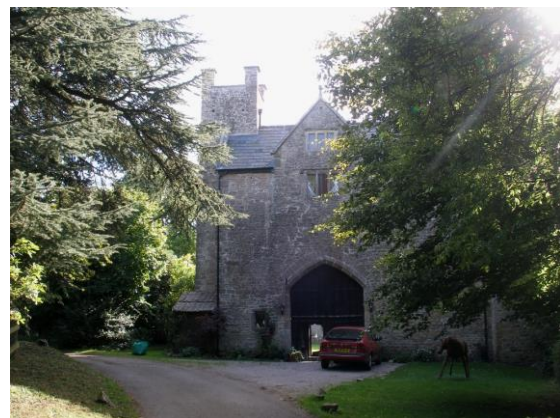
Fig.52 The Gatehouse of Moynes Court, a sturdy medieval structure with a low tudor arch and tower
