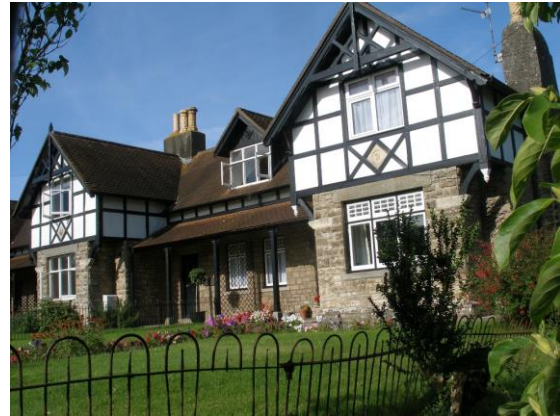
Fig.61 This Domestic Revival terrace of estate cottages has attractive verandas and recalls medieval architecture in its decorative half-timbered gables and mullioned windows
