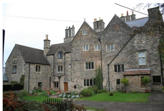
Fig.17 Mullion windows are a striking feature of Moynes Court
