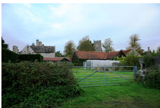
Fig.72 View to the palace with church tower behind
