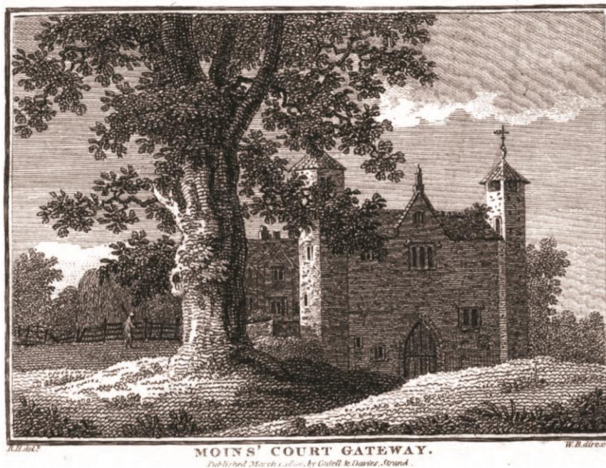
Fig.4 Moynes Court gateway by R.C. Hoare c1800
