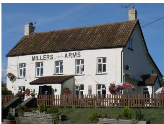
Fig.54 The Millers Arms Inn retains its vernacular character with gable end chimneys and single-storey 'catslide' roof extension to the rear. The large porch is probably a later addition
