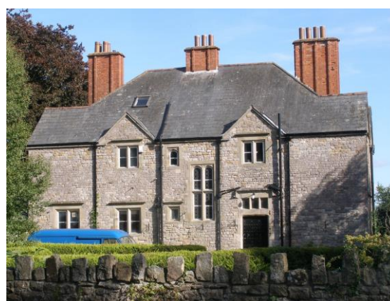
Fig.59 Mathern Vicarage is a powerful, boldly expressed design, enhanced by its massive, incised red brick stacks, a perfect foil to the severity of the stone and slate. Tudor revival drip mould lintels and stone mullions, contrasting with a tall staircase window
