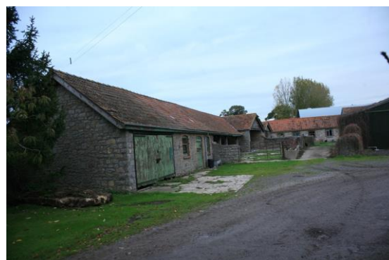
Fig.16 Double Roman interlocking clay tiles are a feature of farm buildings including those at Innage Farm
