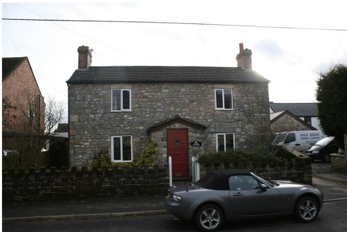
Fig.74 Rose Cottage; Modern roof coverings and modern porch and door have eroded the traditional character of this cottage but these changes are reversible
