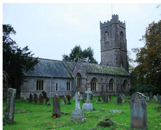
Fig.49 St Tewdric's church. A mainly 14 th century building including a graceful tower. Its relatively large size is due to its relationship to the adjacent Bishops Palace. The church was extensively restored in the 19 th century
