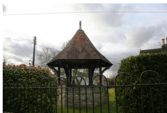
Fig.32 The locally distinctive water tank structure, a key feature within the character area
