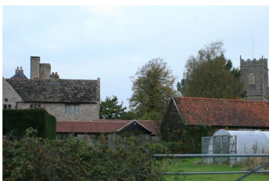
Fig.67 Clay pantiles to Mathern Palace outbuildings
