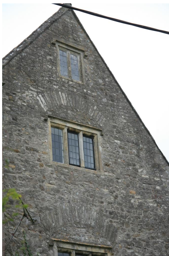
Fig.65 Stone mullion windows to Moynes Court reflecting the higher status of this house
