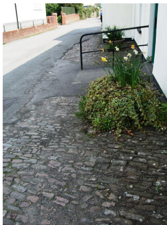
Fig.46 Historic stone setts survive on Brassknocker Street
