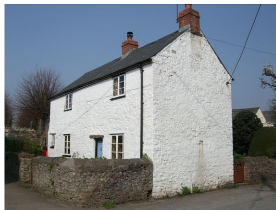
Fig.26 Stone is often white-washed as seen here to the cottage leading to the church
