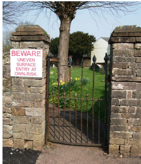
Fig.33 Wrought iron gate to the churchyard
