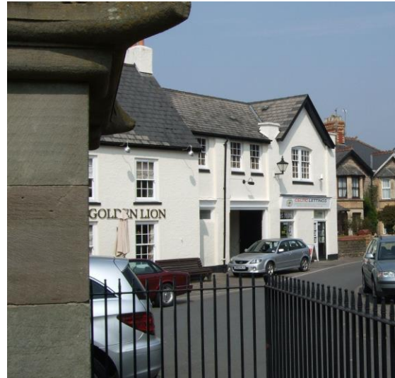
Fig.11 The extension to the Golden Lion retaining the host building's scale and frontage building line
