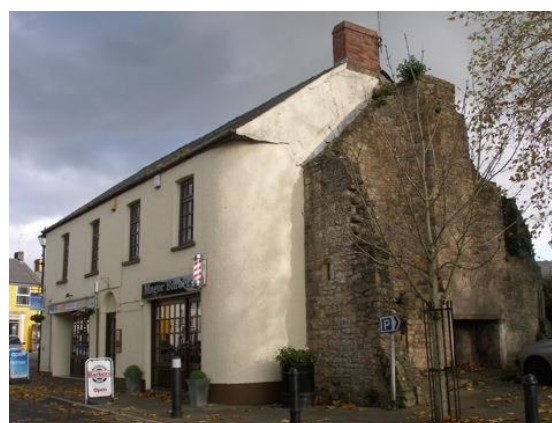
Fig.67 A building of considerable interest. The rounded corner and attachment to the remnants of a late medieval two storey building suggest 17 th century origins.
