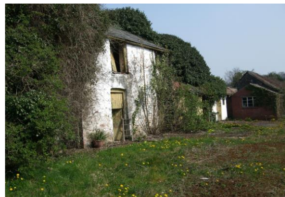
Fig.42 White-washed farm buildings to Manor Farmhouse
