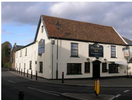
Fig.68 The Wheatsheaf Inn. The low ceilings on the ground floor, steep roof with gable ends and long rear range indicate a building of perhaps 17 th century origins, despite its loss of chimneys and the later windows.
