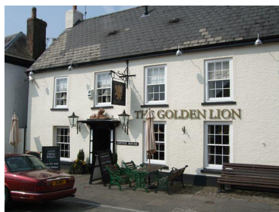
Fig.15 Traditional single glazed timber vertical sliding sashes, the Golden Lion
