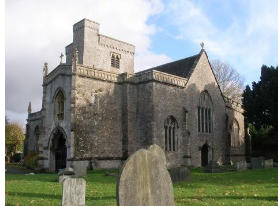
Fig.60 St Mary's Church. The west front, with large mullioned and traceried windows and broad aisles and the two storey late medieval north porch.
