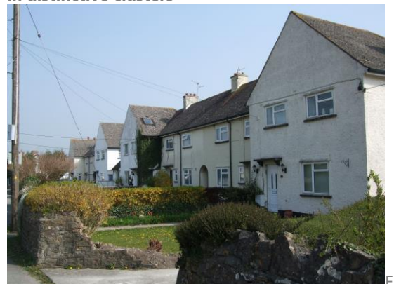
Fig.49 1950s terrace set back from the roadside
