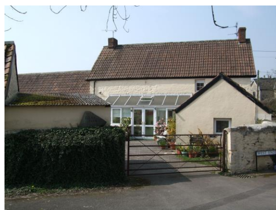
Fig.28 Clay pantiles and Double Roman tiles are a feature of Court Farm
