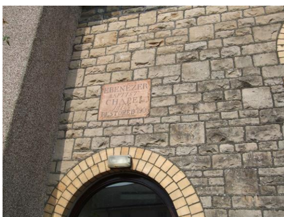
Fig.13 The attractive use of squared stone to the Baptist Chapel used in conjunction with yellow brick dressings
