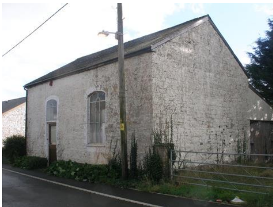
Fig.77 Former Chapel, West End. This vacant building, although extended and in need of sensitive conservation, is a physical reminder of the heritage of Magor, for both its original purpose and simple design.
