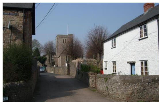
Fig.23 Built form defines a pinch point in the townscape creating a well-defined route through to the parish church and old school
