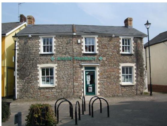
Fig.12 The pharmacy is constructed in rubblestone, one of a number of traditional local materials seen in this part of the Conservation Area
