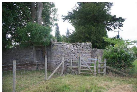
Fig.9 Llantilio Court's boundary walls survive as reminders of the scale and extent of the former house and grounds
