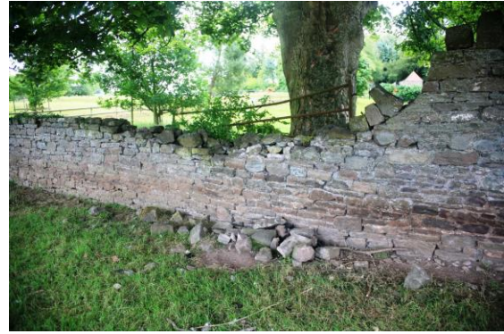
Fig.15 Coursed sandstone rubble walls are a feature of the former Court grounds
