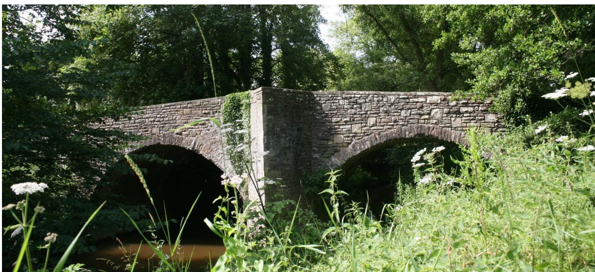
Fig.43 The stone bridge is a local feature of historic and architectural significance and forms part of the eastern approach to the village
