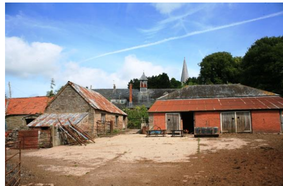
Fig.17 Agricultural buildings at Court Farm display a wide variety of materials including rubblestone, brick, clay tile, slate and corrugated iron
