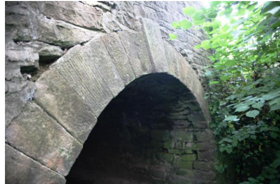
Fig.22 19 th century stone bridges take roads over the White Castle Brook
