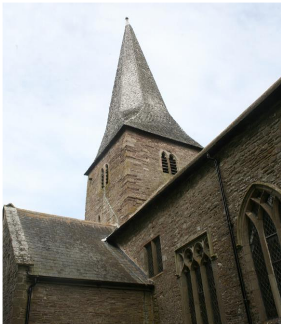
Fig.14 The sandstone church exhibits a fine shingle spire
