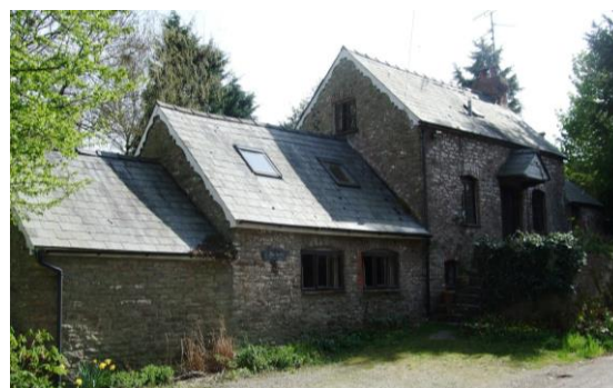
Fig.30 The Blacksmiths is set on the roadside
