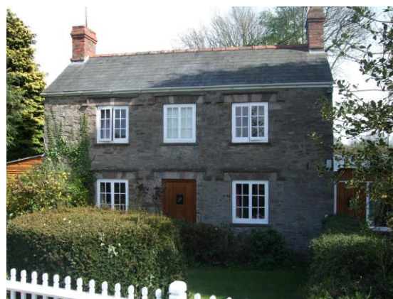
Fig.36 Hostry Cottage displaying sandstone rubblestone and ashlar dressings
