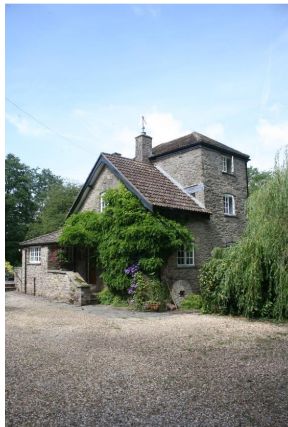
Fig.56 Former Water Mill. Originally the tower was slightly higher and had a, presumably, Victorian timber-framed top storey. The building has been converted to residential use
