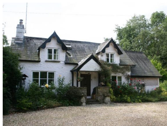
Fig.46 Cottage near the former Water Mill. Its basic form is that of a vernacular dwelling although it appears to have been adorned with later Victorian additions including the decorative bargeboards
