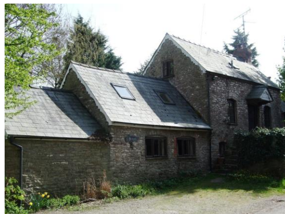
Fig.44 Former Blacksmiths. A typical vernacular composition of main building and secondary wings set out in linear fashion and of diminishing heights.
