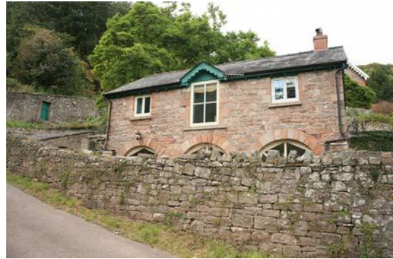
Fig.45 Rubblestone boundary wall
