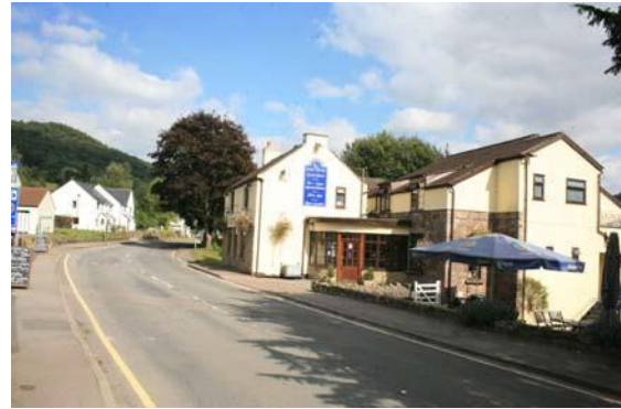
Fig.40 The Sloop Inn - a prominent building in views along the A466
