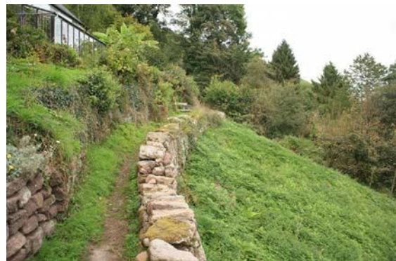
Fig.31 Footpaths are often demarcated by stone walls
