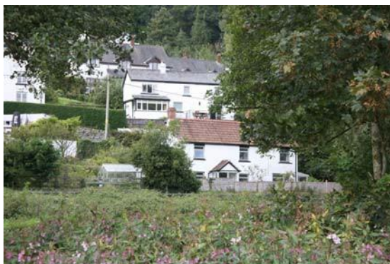
Fig.13 Hillside development in Llandogo displaying the usual painted rendered finish and a mix of slates and tiles to roofs
