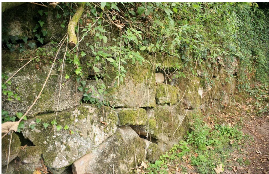
Fig.25 Dry stone walls are a defining local feature of the Conservation Area
