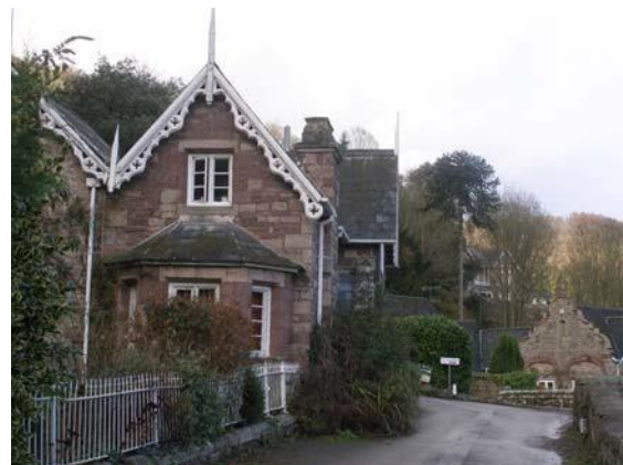
Fig.38 The Flemish gable of the stables to The Priory seen in the distance
