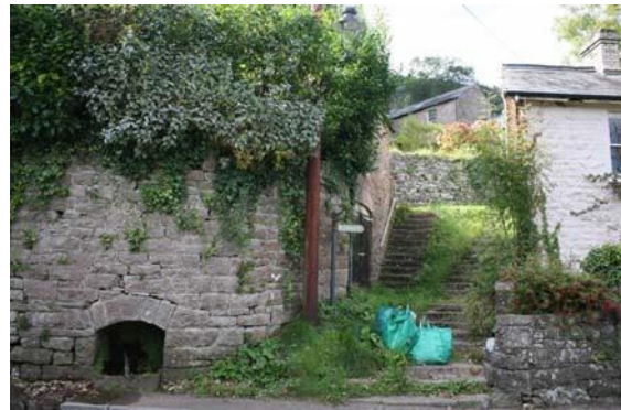
Fig.46 Stone steps & stream culvert
