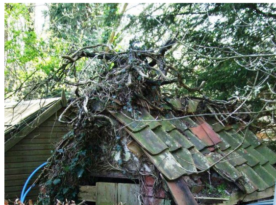
Figure 33 Clay pantiles are found on many outbuildings including this small building in the grounds of The Old Victoria
