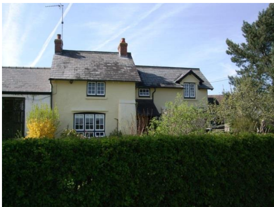
Figure 31 School House with traditional natural slate roof
