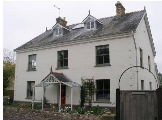
Figure 63 Holmer House. The simple symmetry of this substantial Edwardian house is enlivened by decorative bargeboards to the dormers and porch, the ornamental ridge tiles and finials and the patterned brickwork of the chimneys.
