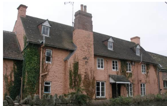
Figure 51 Church Farm (formerly The Pentre) dates from the 17 th century, as indicated by its long narrow form, steep roofs and massive lateral chimney.
