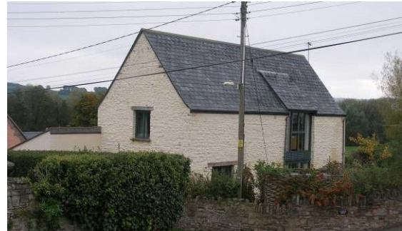
Figure 53 Willow Barn. This sensitively converted barn, part of the Church Farm/ Village Farm complex retains most of its original features.
