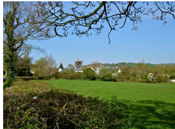
Figure 72 View of the church tower from the north
