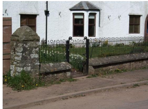
Figure 35 Historic iron railings and gate at the Old Vicarage
