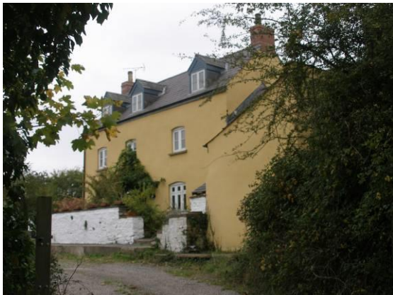
Figure 58 Rock Farm House looks towards Llandenny from the west of the conservation area. This tall well-preserved early 19 th century farmhouse presides over a farmyard enclosed by important examples of traditional farm buildings.
