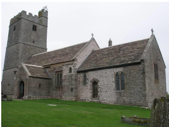
Figure 50 St John's Church from the south-east. The building has Norman origins, but its elegant tapering tower, seen from many vantage points dates from the 15 th century.
