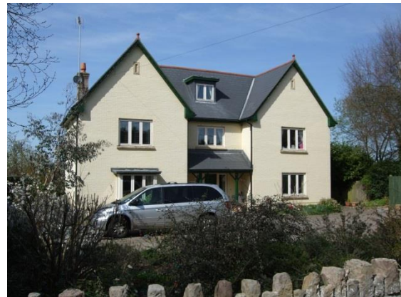
Figure 64 Rumpus House. A recent house inspired by Victorian domestic precedents. Its recessed location behind the stone boundary wall defers to its established neighbours.
