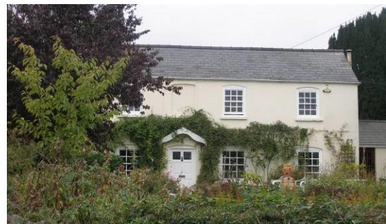
Figure 54 The Elms retains a full set of 18 th century sash windows on its regularly proportioned front elevation.
