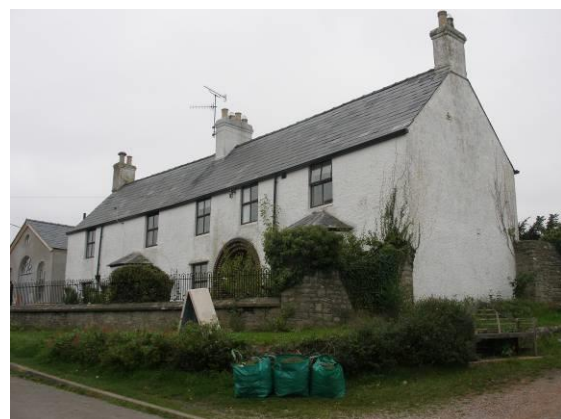
Figure 49 The former vicarage, a vernacular building, altered with Victorian and 20 th century additions.
