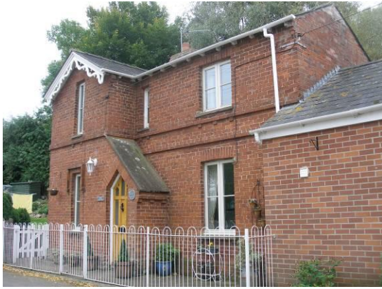
Figure 57 Brick Cottage. An inventive asymmetrical design for this modest Victorian house uses interesting brickwork detailing. The single storey element is a later addition.
