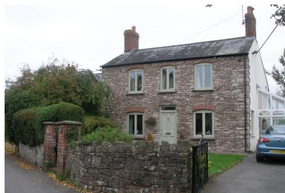
Figure 62 The Ferns. An attractive 19 th century cottage, standing behind original cast iron gates. Its red brick voussoirs contrast well with the rubble stone walls. The well-designed timber casement windows are probably replacements.
