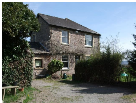
Figure 34 Historic sash windows survive at Oakfield
