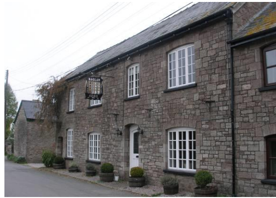
Figure 60 The Raglan Arms. The flush façade and regularity of fenestration is enhanced by the fine detailing of its stonework, especially in the 'random' coursing and dressings and well executed cambered stone window heads.
