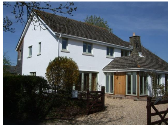
Figure 67 The rendered and weatherboarded Oakways
