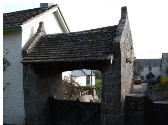
Figure 68 The lych gate, one of only three structures with stone tile roofs
