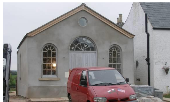
Figure 56 The former Victorian, non-conformist chapel, substantially rebuilt and converted. The simplified classical symmetry is typical of this building type.
