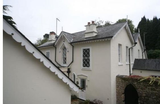
Fig.109 Ashfield with picturesque styling to window openings and bargeboards
