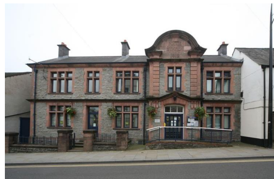
Fig.78 The rock-faced stone Police Station (1912)
