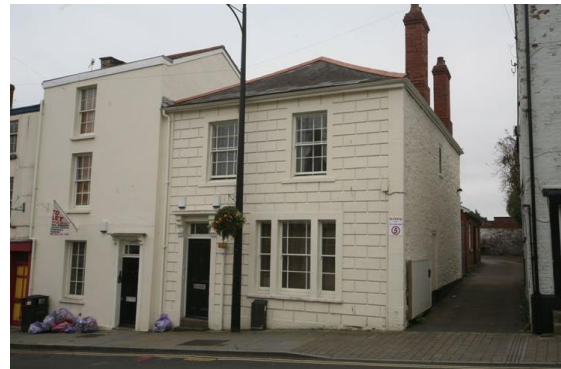
Fig.75 No. 3 Moor Street with its distinctive and somewhat unusual stucco façade on a building of this scale
