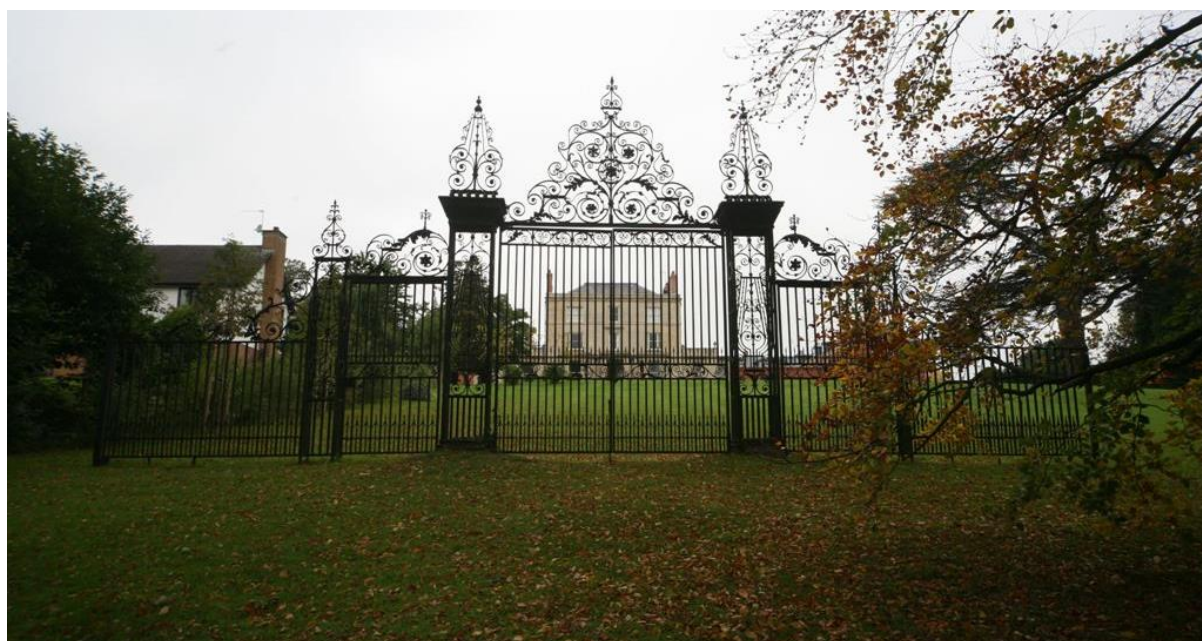
Fig.89 The well executed and highly decorated Grade II listed gates to The Mount
