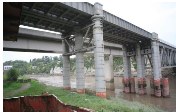
Fig.57 Brunel's railway bridge
