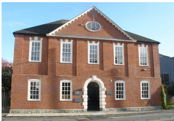
Fig.129 Picton House, 1907 Lower Church Street. Its bold pediment with elegant oval window sits over a regular but rather unusual 18 th century style façade.
