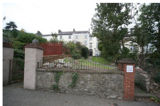
Fig.90 The 1832 development of Mount Pleasant terrace enjoys views east to the River Wye
