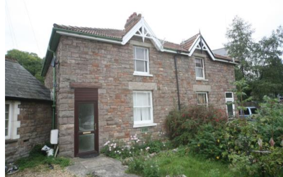
Fig.64 The Quarries feature squared stone
