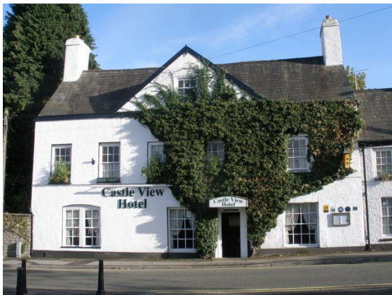
Fig.127 Castle View Hotel: 18 th century with characteristic Chepstow gable, plus Georgian sashes.
