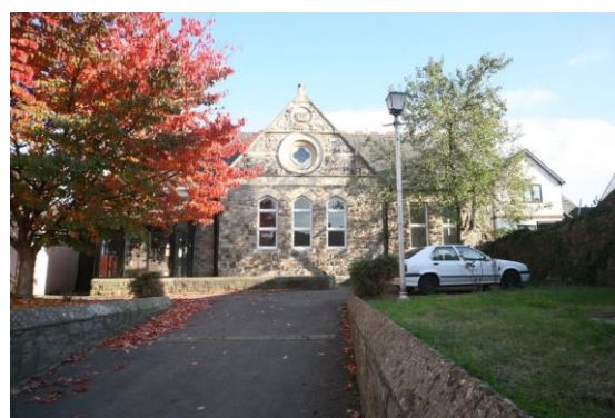
Fig.29 Occasional buildings such as the former Chepstow Board School are set back from the roadside interrupting the generally strongly defined and consistent building line
