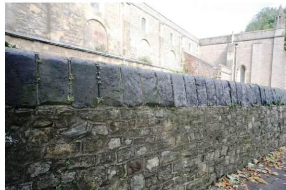
Fig.162 Slag blocks used as copings to the churchyard wall
