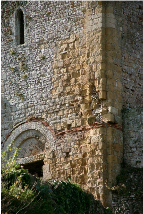
Fig.45 Large blocks of yellow Triassic sandstone are seen here with Roman tiles
