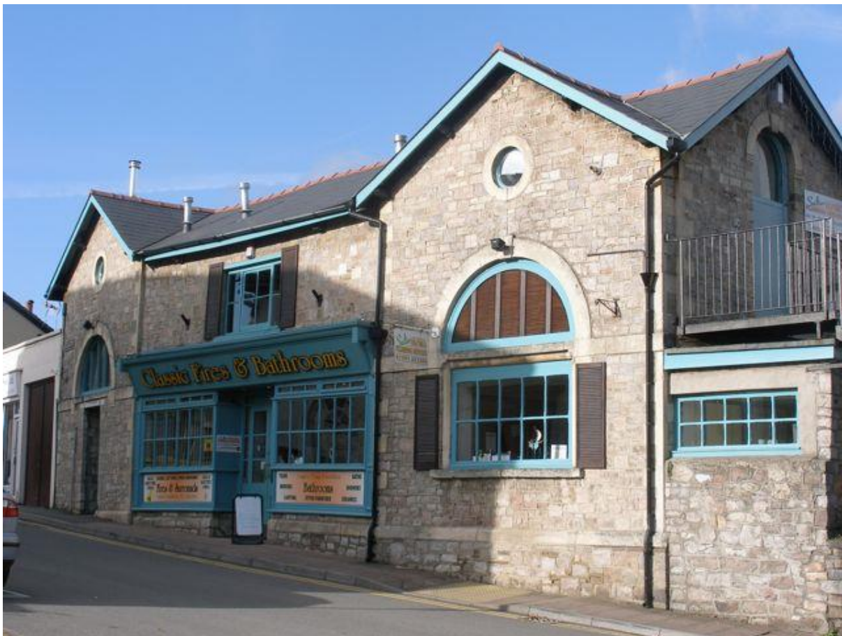
Fig.144 Shop, Station Road. Italianate design principles enhance this functional mid-19 th century commercial building.
