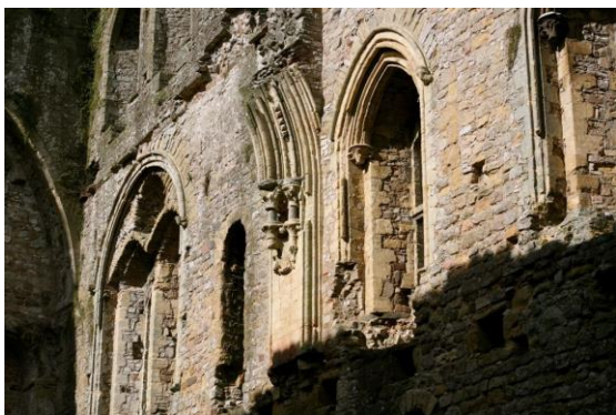
Fig.46 Devonian sandstone and carboniferous limestone are used in conjunction in the Great Tower
