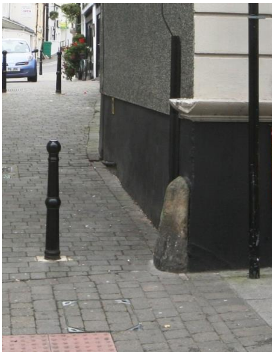
Fig.83 Stone buffers featured on buildings were used to protect buildings from being struck by wagon wheel hubs.
