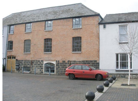
Fig.138 Warehouse adjacent to Wye House. The plinth is constructed of furnace slag blocks.
