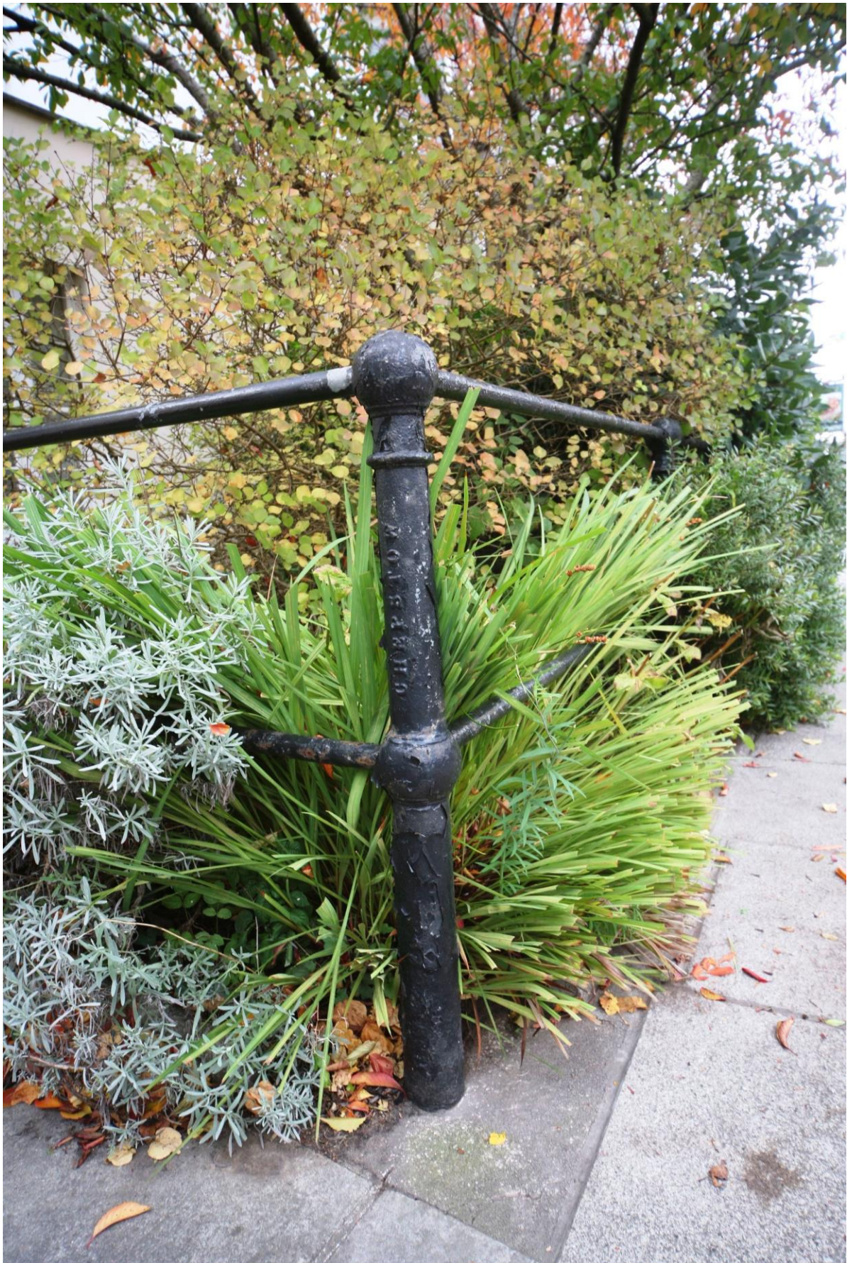
Fig.84 Railings bearing Chepstow foundry marks are a local feature
