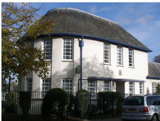
Fig.151 Job Centre Plus. A well preserved and rare example of 1930s modernism in the town, although the steep pitched roof recalls earlier periods.
