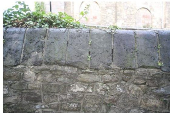
Fig.33 Slag blocks are a feature of special note
