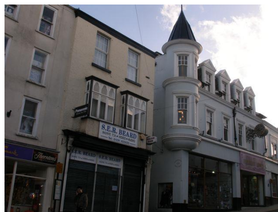
Fig.146 Coronation Buildings 1902. The 'pepperpot' pinnacled corner turret makes a positive contribution to the skyline of the High Street.
