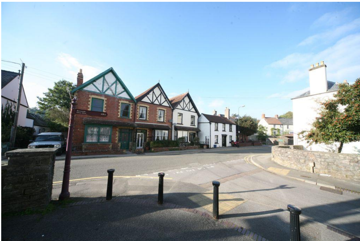
Fig.34 Contrasting character of Nos 1-2 Bridge Street with brick frontages and timbered gables
