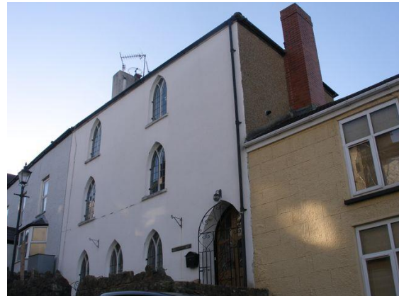
Fig.135 Hawkpoint in Steep Street. Another example of 'Gothick' windows used in a basically Georgian house.
