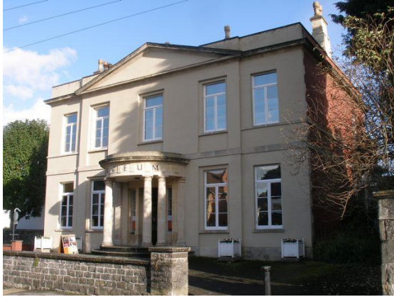
Fig.132 Gwy House, the Chepstow Museum; a refined Palladian style house with correct Tuscan columns supporting a semi circular portico.
