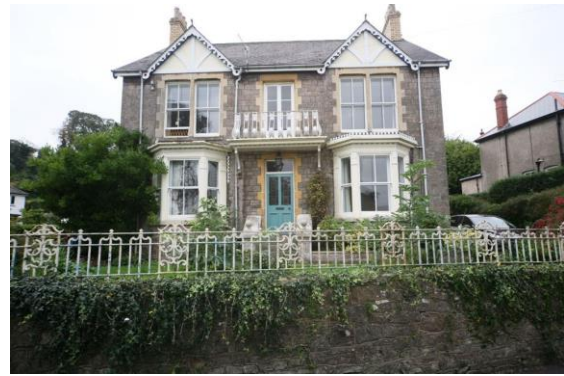
Fig.98 The late Victorian villa of Stoneleigh has fine examples of timber detailing and ironwork
