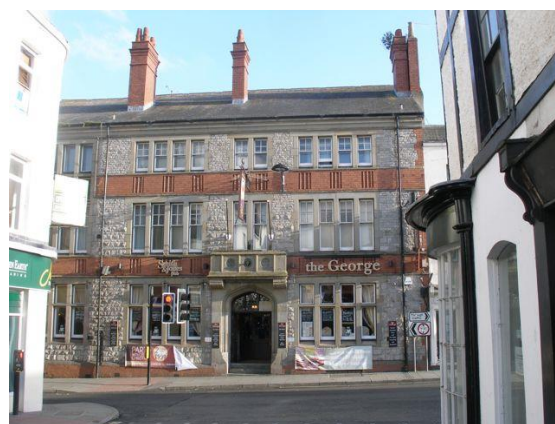
Fig.147 The George Hotel uses mullions and contrasting bands of brick and stone in an almost modern manner.
