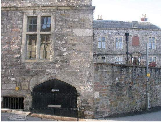
Fig.126 The Powis Almshouses, built in 1716, a hybrid containing Queen Anne classicism, but also incorporating earlier stylistic features into the design.
