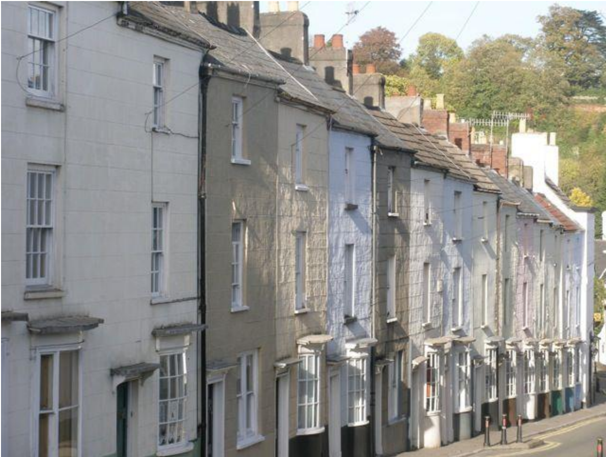
Fig.136 Castle terrace. This regular Regency terrace with its characteristic subtle bow windows is one of the memorable images of Chepstow.
