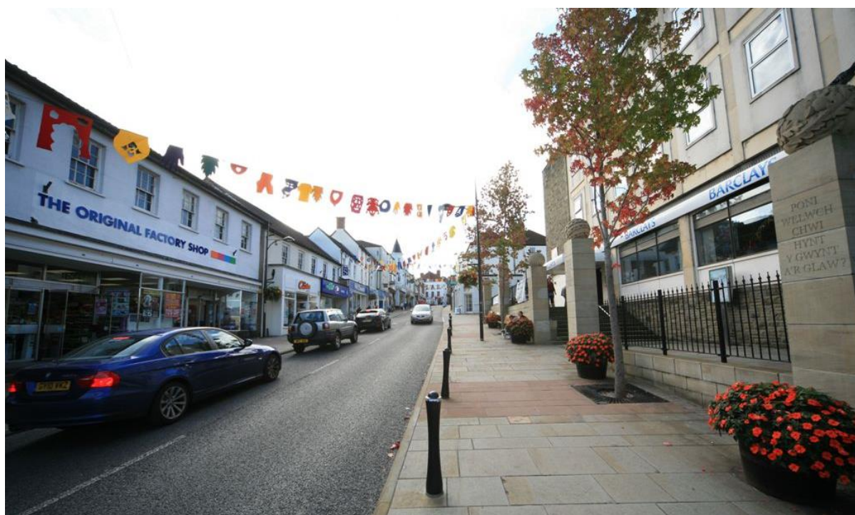
Fig.14 The High Street has a strong building line with shops to the back of pavement
