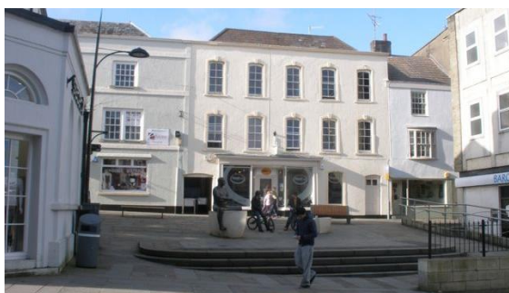
Fig.131 Nos. 6 and 7 Beaufort Square, with early 18 th century window surrounds, is a broad fronted town house, altered for commercial uses on the ground floor.
