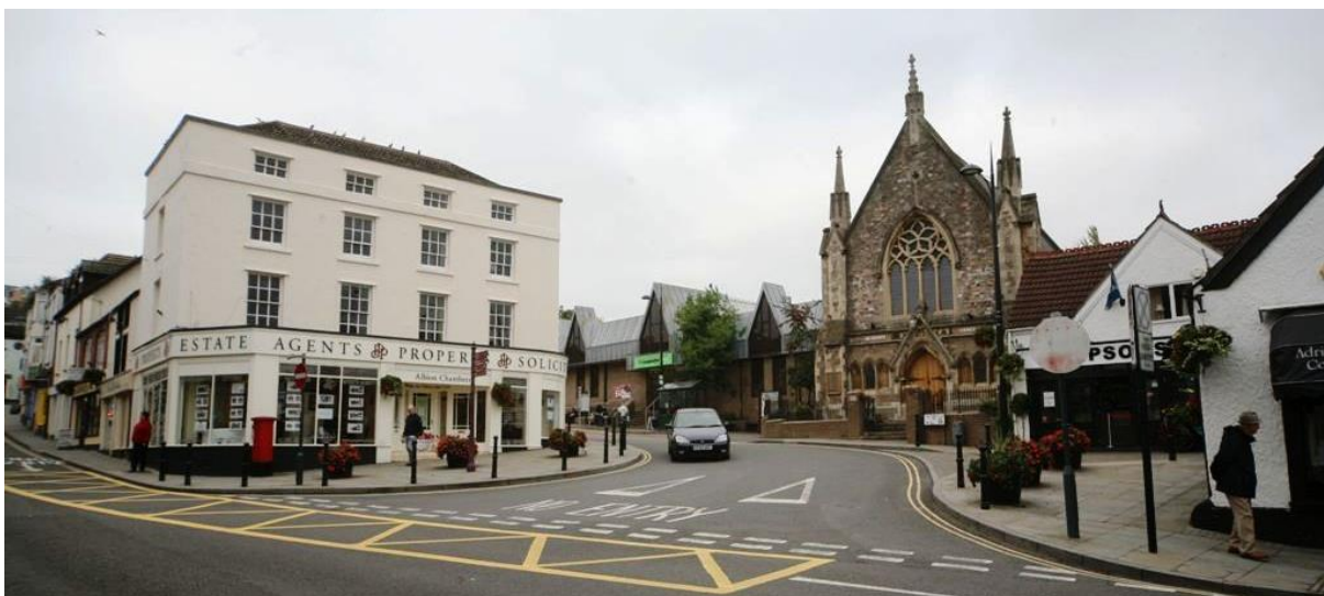
Fig.70 Albion Square, showing impact of traffic management at the junction
