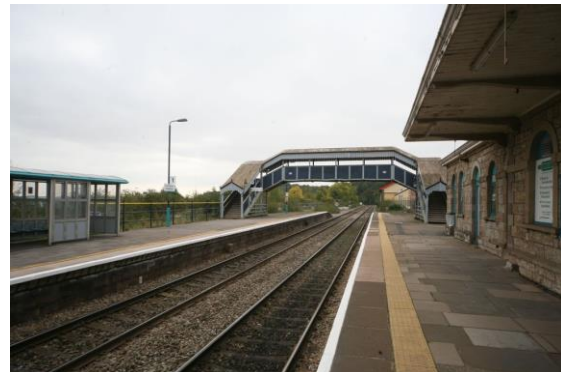
Fig.62 The 1892 cast iron footbridge
