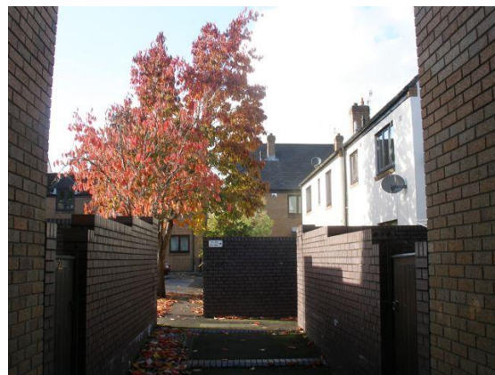
Fig.153 Hollins Court, a successful infill scheme which received a housing award in 1985, creates an intimate network of lanes and 'places'.
