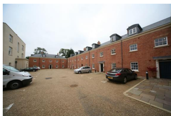
Fig.87 The rear courtyard of The Mount with a range of new red brick buildings
