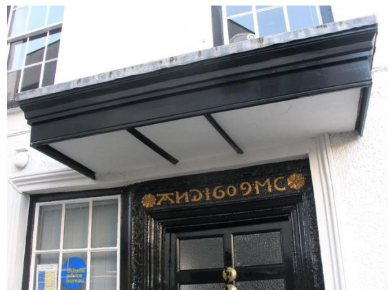
Fig.124 The Gate House, this early Stuart carved doorway is absorbed into the 18 th century refronting of the house.
