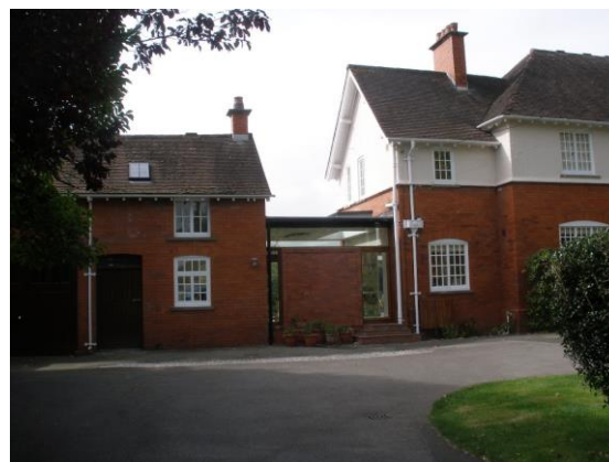
Fig.58 Coach houses and stables are valuable survivals – this image shows a sensitive intervention to link the house with its outbuildings without compromising the integrity of either building
