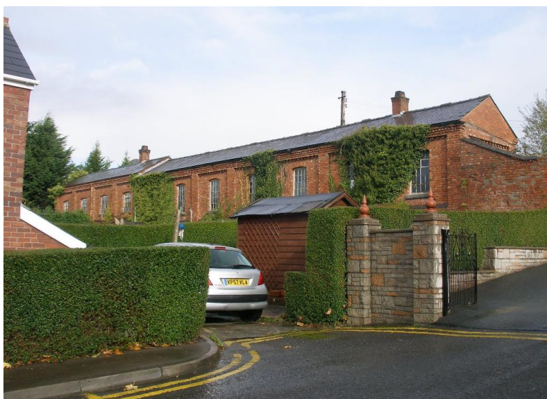
Fig.68 The Goods Building – a long brick range equivalent to two storeys in places (here seen from Hatherleigh Rd)
