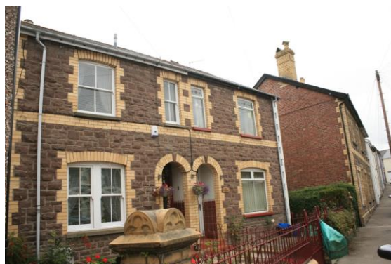
Fig.59 A typical combination of materials seen throughout the conservation area – Pennant Sandstone laid to courses with brick dressings to windows, doors and string course
