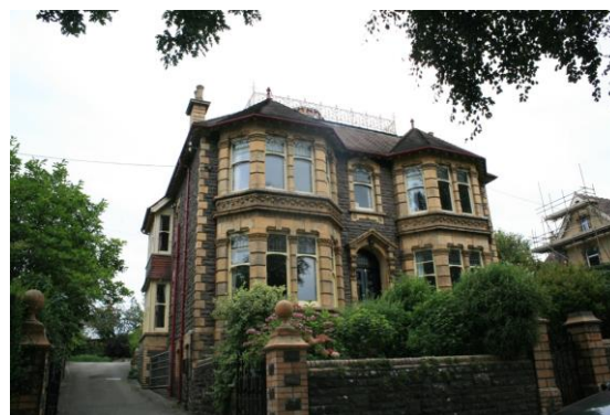
Fig.12 An eclectic mix of building materials to the villas in this part of the conservation area
