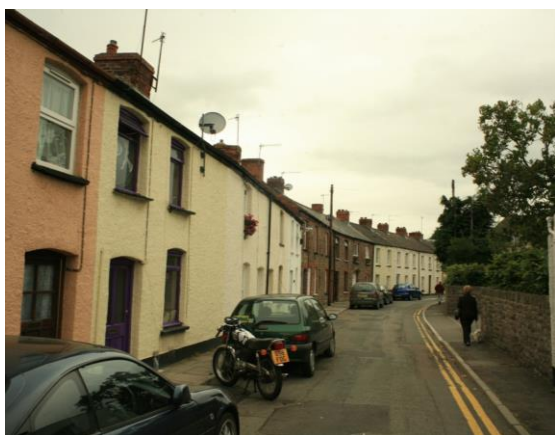
Fig.53 A mix of painted render and stone facades with slate roofs and brick chimneys characterises much of the high density Victorian housing in Abergavenny
