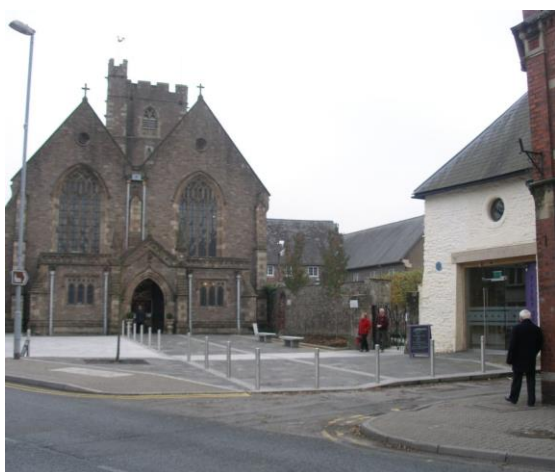
Fig.39 The church of St Mary within its recently refurbished public realm setting
