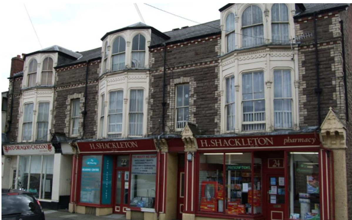
Fig.29 A rich palette of traditional materials is seen in this part of the conservation area (shops with accommodation above, Brecon Rd)
