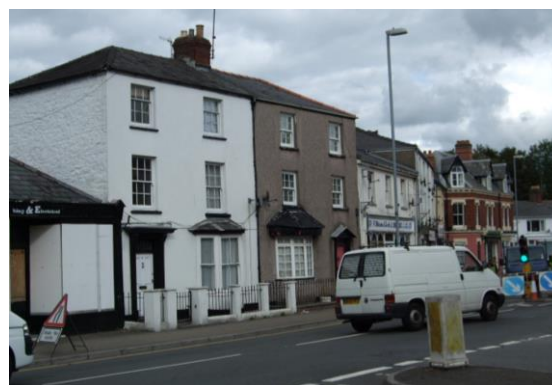
Fig.55 North side of Brecon Rd nr junction with Frogmore St – an attractive group of unlisted buildings; shops, offices, houses and flats
