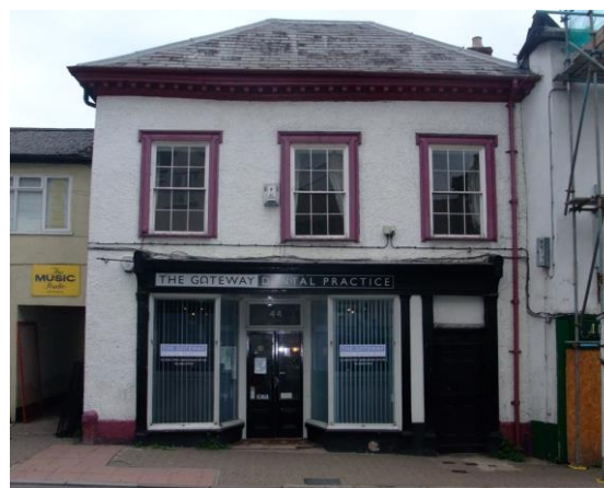
Fig.20 Good quality 19 th century shopfront, with side-entrance and 12-pane vertical sliding timber sashes (a common feature of the historic core)
