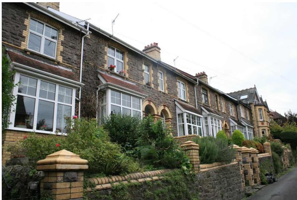
Fig.13 Stone boundary walls with buff brick copings are key features of this part of the conservation area
