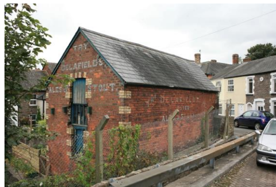
Fig.25 Traditional painted signage to walls surviving on an outbuilding off Union Road East
