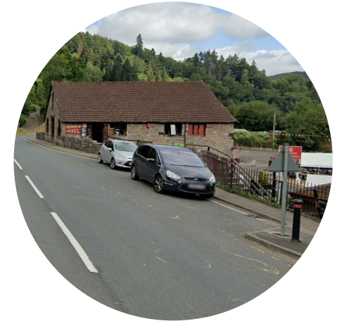
Narrow footway associated with on-street parking, Tintern
