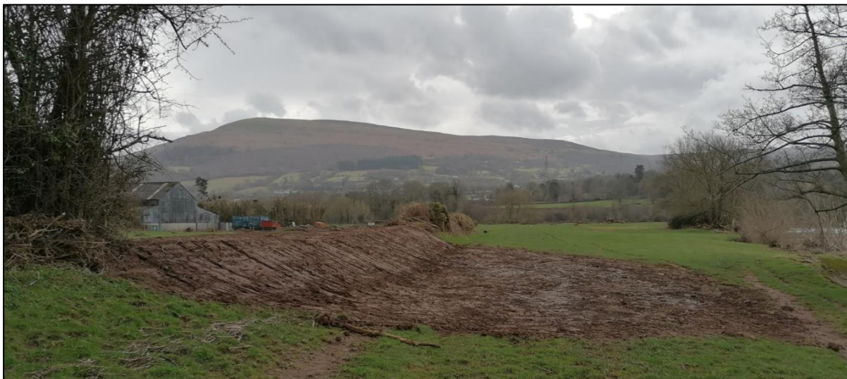
Photo 5: Part of the reinstated embankment on 7 th March 2020.
