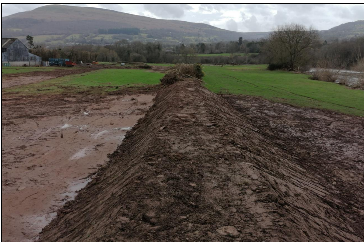
Photo 6: Part of the reinstated embankment on 7 th March 2020.
