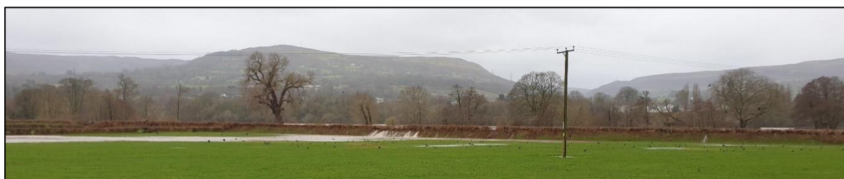
Photo 4: Overtopping of the northern part of the flood embankment continuing at 11:52 am on Sunday 16 th February 2020.
