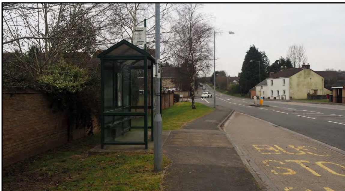
Photograph 19: Westbound Bus Stop Serving the Development Site
