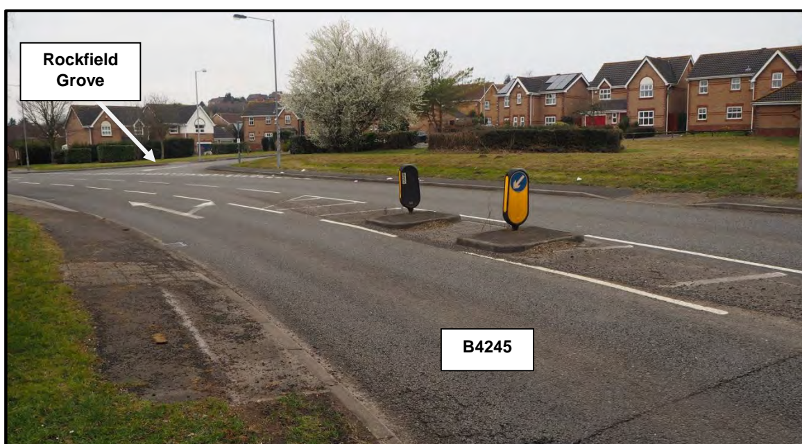
Photograph 16: B4245 adjacent Rockfield Grove (looking west)
