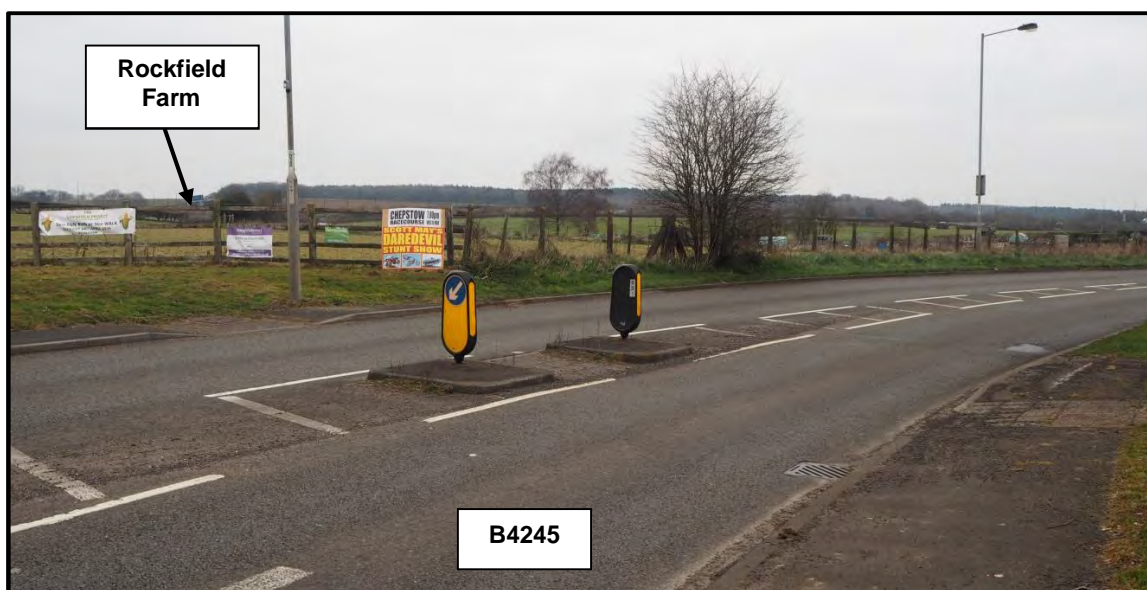
Photograph 15: B4245 adjacent Rockfield Grove (looking east)
