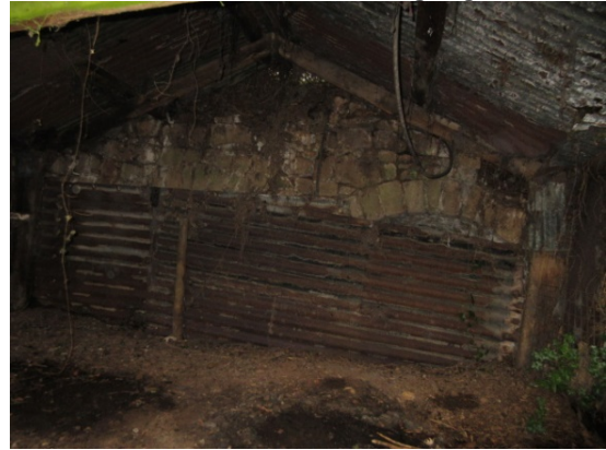
Plate 18: South-west end wall of the garage
