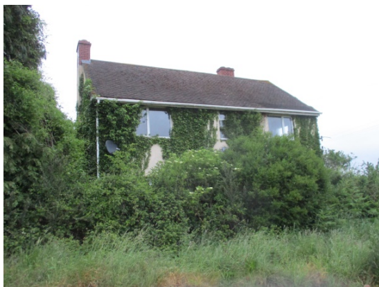
Plate 20: South elevation of House
