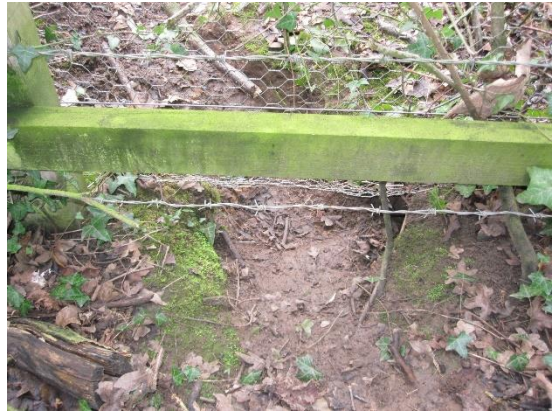
Plate 4: Typical failure of badger proof fencing noted on both sides of the M4
