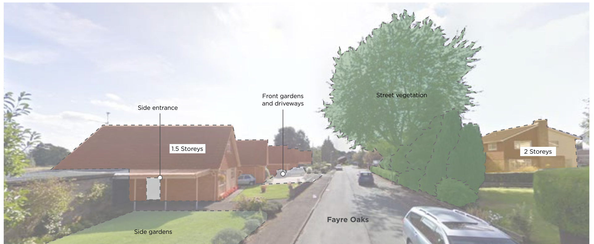
Varying building heights and landscape treatment along Fayre Oaks
